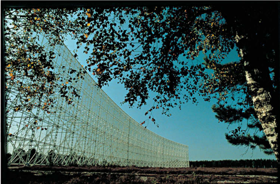
The spherical reflector of the great radio telescope at Nançay, in the Sologne region of France. This instrument can be used to transmit or receive radio signals as part of the search for extraterrestrial civilisations.
