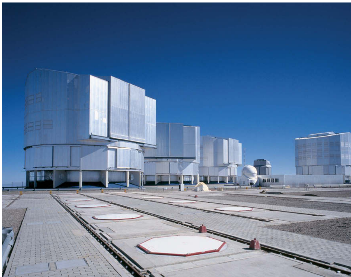
The VLTi interferometer at Paranal Observatory, Chile. This photograph, taken in March 2005, shows the four 8.2-metre telescopes of the ESO's Very Large Telescope (VLT). The VLTi is able to link these instruments, and three auxiliary telescopes, together as an interferometer.
