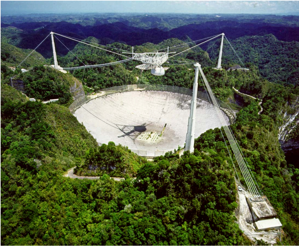
FIGURE 14.5 The 305 meter dish of the Arecibo radiotelescope in Puerto Rico. (Photo courtesy of the NAIC-Arecibo Observatory, a facility of the NSF. Photo by Tony Acevedo)
