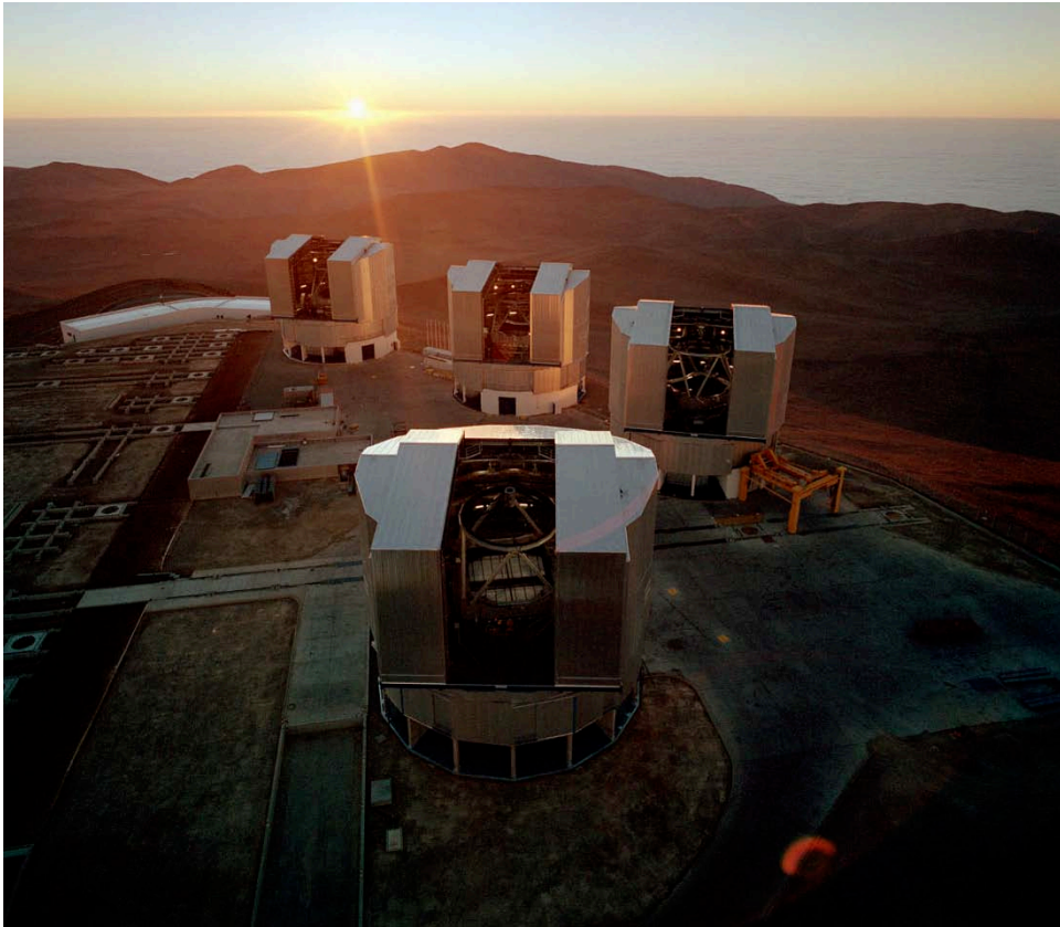
FIGURE 8.5 The European Southern Observatory's VLT group of telescopes at an altitude of 2640 meters on Cerro Paranal in Chile. The four largest each has an aperture of 8.2 meters. (ESO, PR photo 43a/99)
