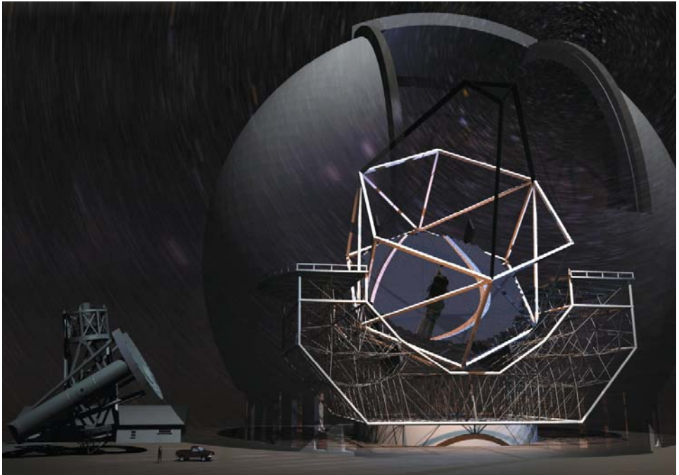
Figure 12.2. Artist's renderings of the TMT and comparison with the Palomar 5-m Hale telescope. This telescope, developed in partnership between the U.S.A. and Canadian institutes, should be available in 2014. Because of the large size of its aperture, combined with the capabilities of AO systems, it will provide an unprecedented spatial resolution of Io, better than most of the Galileo spacecraft infrared observations (courtesy California Institute of Technology).
