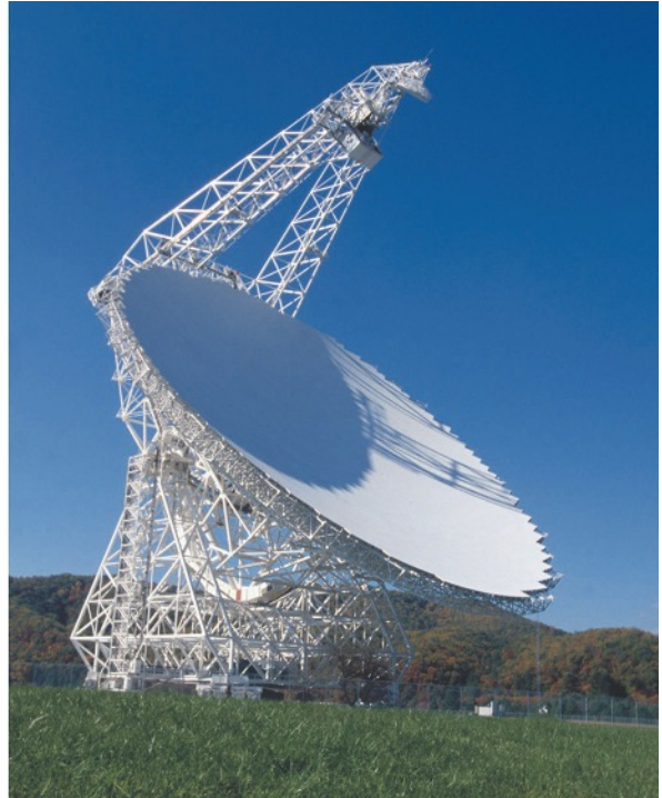
are necessary for this. Right: The Green Bank Telescope. It does not have a rotationally symmetric mirror; one axis has a diameter of 100 m and the other 110 m
