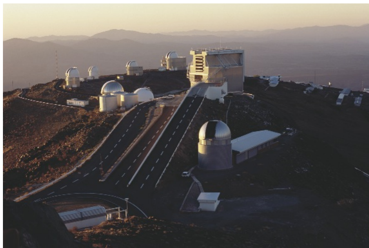
Fig. 1.26. The La Silla Observatory of ESO in Chile. On the peak in the middle, one can see the New Technology Telescope (NTT), a 3.5-m prototype of the VLT. The silvery shining dome to its left is the MPG/ESO 2.2-m telescope that is currently equipped with the Wide-Field Imager, a 8096^2 pixel camera with a 0.5^\circ field-of-view. The picture was taken from the location of the 3.6-m telescope, the largest on La Silla
