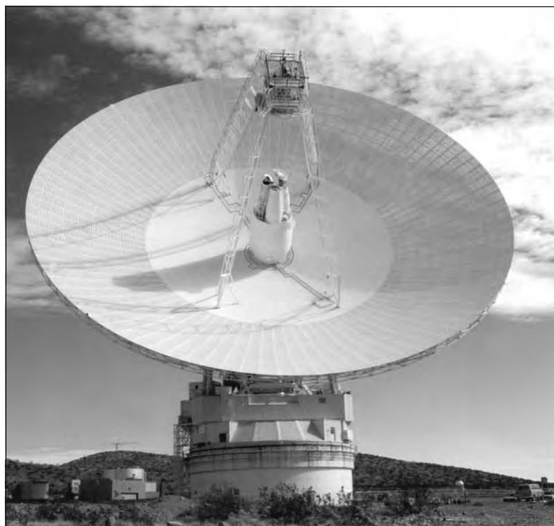
One of several radio dishes located at the Goldstone complex in the Mojave Desert of California. These sensitive paraboloid dishes can be moved to face incoming radio waves, which are reflected to a subreflector located in the housing at the top of the four scaffold-like towers (center), which in turn beams these concentrated waves through a feed horn in the center of the dish and down to a control room where a receiver amplifies the signals and computers render them into images. (NASA)
