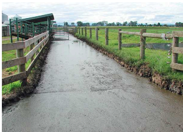
Figure 8-5 Trackways that are lower than the surrounding land become exceptionally muddy. (Courtesy of J Malmo)
