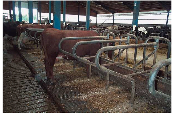
Figure 6-16 A spacious barn with a central feed truck alley between two rows of feed stalls with individual stall partitions and rubber flooring. (Courtesy of C Bergsten)
