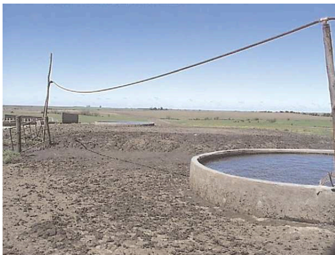
Figure 9-1 Although this watering station provides good perimeter access, it is too low to the ground; the perimeter around is very muddy and should have a concrete apron. (Courtesy of R Acuña)
