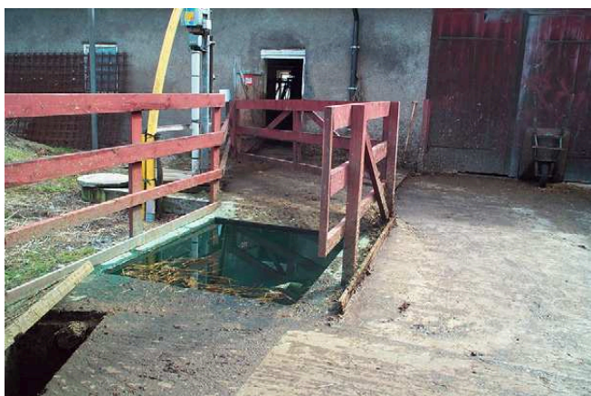
Figure 14-31 This foot bath is located in the open and is not sufficiently long to provide good service. (Courtesy of C Bergsten)
