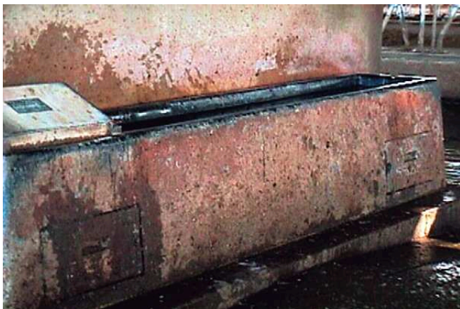
Figure 9-6 This water trough is too deep and has no drainage plug. It will inevitably become heavily contaminated with debris and bacteria. (Courtesy of R Shaver)
