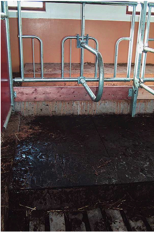
Figure 6-14 An individual feeding stall with rubber mats and a short partition. (Courtesy of C Bergsten)
