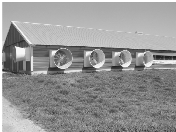
Fig. 3 Tunnel fan end of commercial house, where 48 inch cone fans are used to move air down and out of the house. This particular house is curtain sided and has a pocket at the top of the curtain opening to allow for a tight seal during brooding and tunnel ventilation. (View this art in color at www.dekker.com .)
