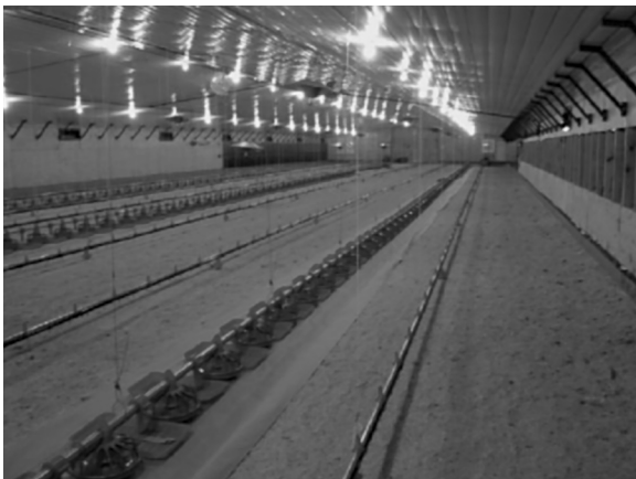
Fig. 2 Commercial broiler house prior to chick placement. Water lines, feed lines, radiant brooders, circulation fans, exhaust fans, and air inlets can be observed. (View this art in color at www.dekker.com .)
