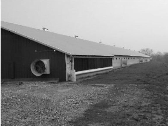
Fig. 1 Tunnel inlet end of a commercial broiler house. Evaporative cooling system, air inlets, and 36 inch exhaust fans can be seen. (View this art in color at www.dekker.com .)
