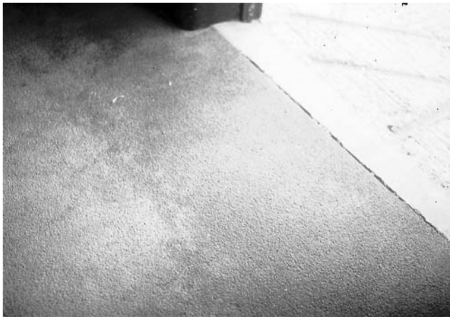
Fig. 15.2. Rubber matting as a flooring for foaling boxes is becoming increasingly popular. It is dust-free and warm and can easily be hosed down and disinfected.
