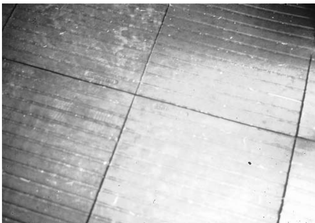
Fig. 13.19. Rubber matting may also be used as a suitable, clean, dust-free, non-slip surface in a covering yard.
