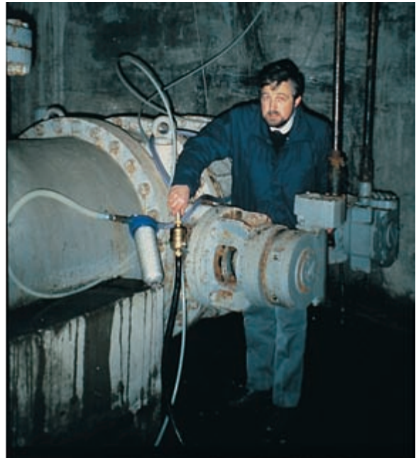
Figure 8.18 Leakage from this drainage system contaminated a public swimming pool, causing a large outbreak of cryptosporidiosis. Courtesy of Dr David Casemore.
