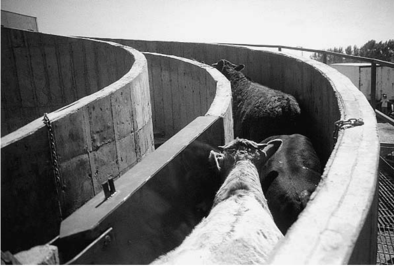
Fig. 20.5. Curved cattle race with solid sides at a slaughter plant.
