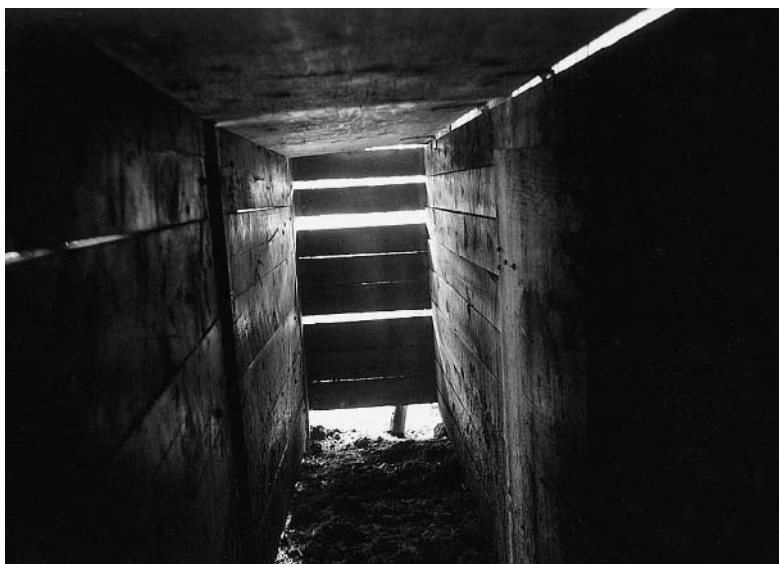
Fig. 7.9. A cow's-eye view into a well-designed dark box. Light slits attract the cow in. In some facilities the slits are covered after the cow is in the box.
