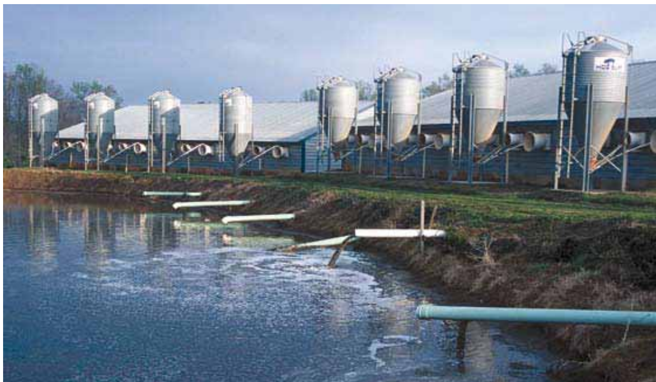
State of the art lagoon waste management system for a 900 head hog farm. The facility is completely automated and temperature controlled – United States 2002
