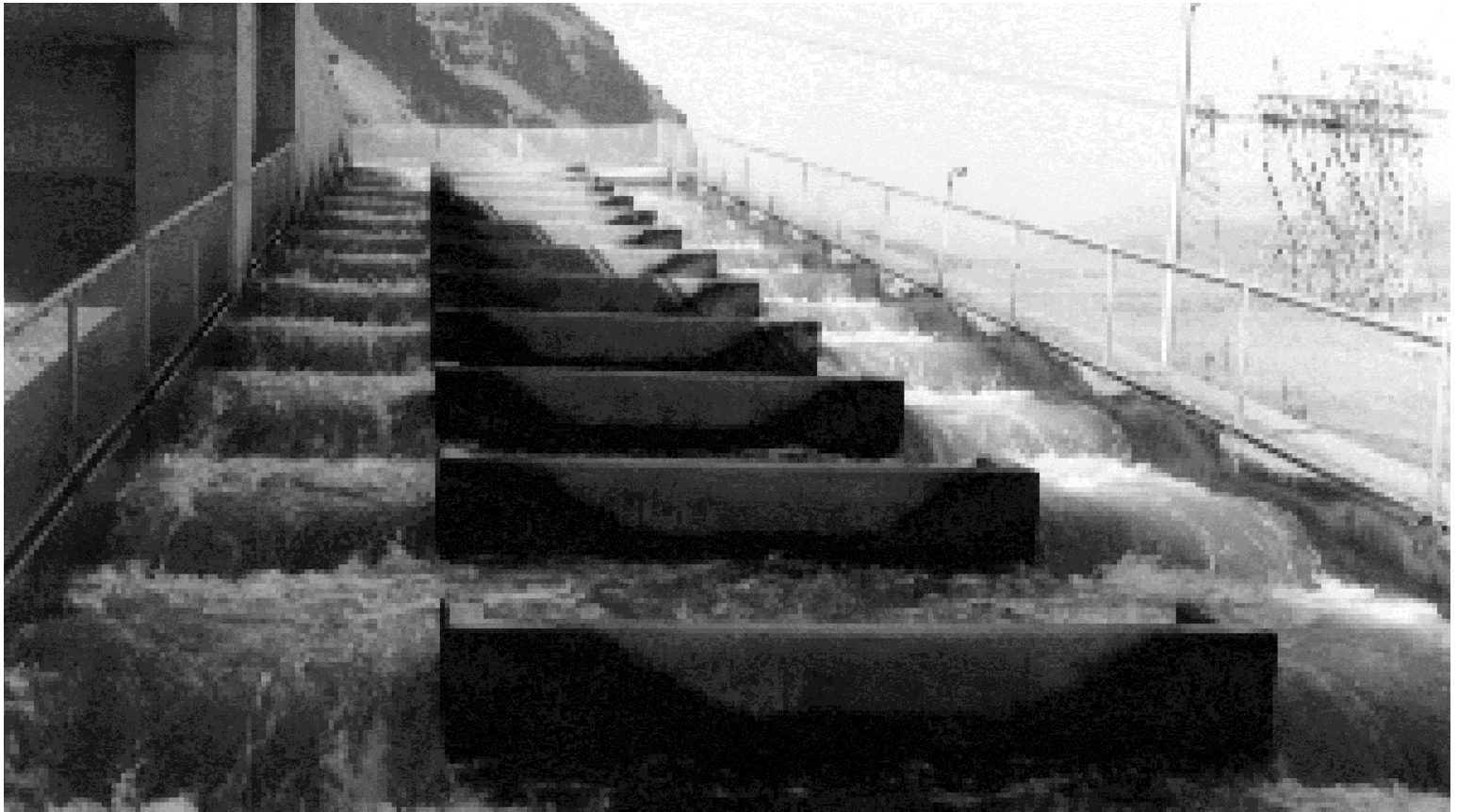
Figure 19–7 Fish ladders provide an opportunity for salmon to return to their birth site and spawn.
