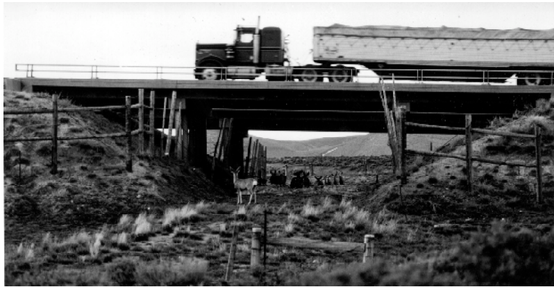
Figure 9–13 Deer fence and underpass prevent deer from entering highway. (Courtesy of L. Ward.)
