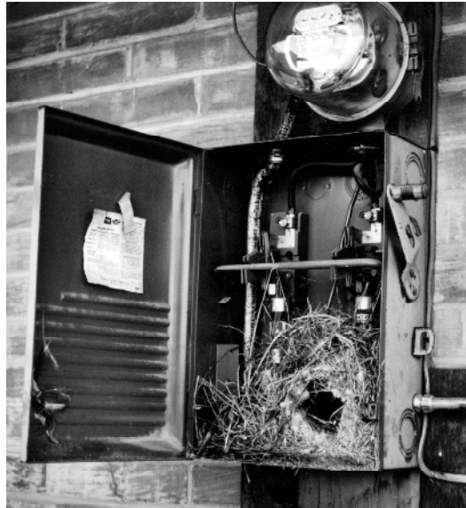
Figure 22–2 House sparrows frequently build their nests in unwanted places. (Courtesy of C. A. Morgan.)
