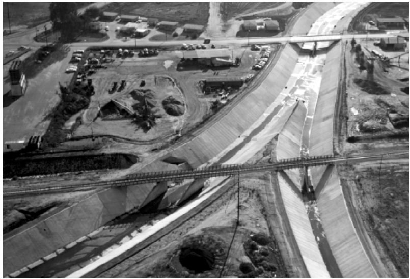
Figure 8–8 Concrete-lined stream channel in an industrial area. (Courtesy of the U.S. Soil Conservation Service.)
