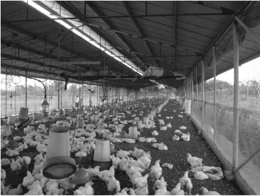
Fig. 5.6. Ridge vent in uninsulated poultry house.
