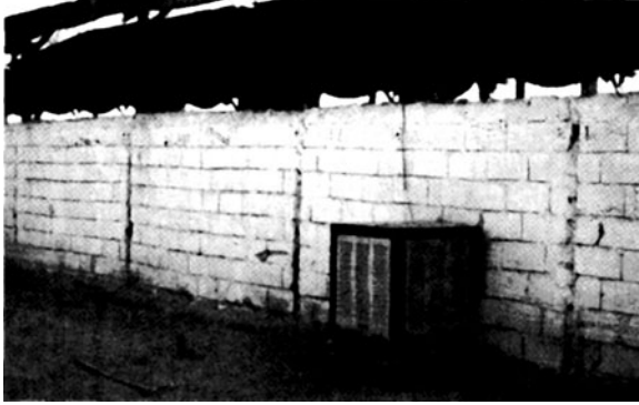
Fig. 9.2. Naturally ventilated house equipped with desert-type air cooler.
