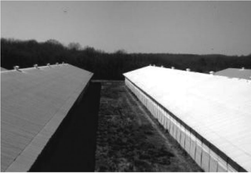
Fig. 5.10. Reflective roof coating.
