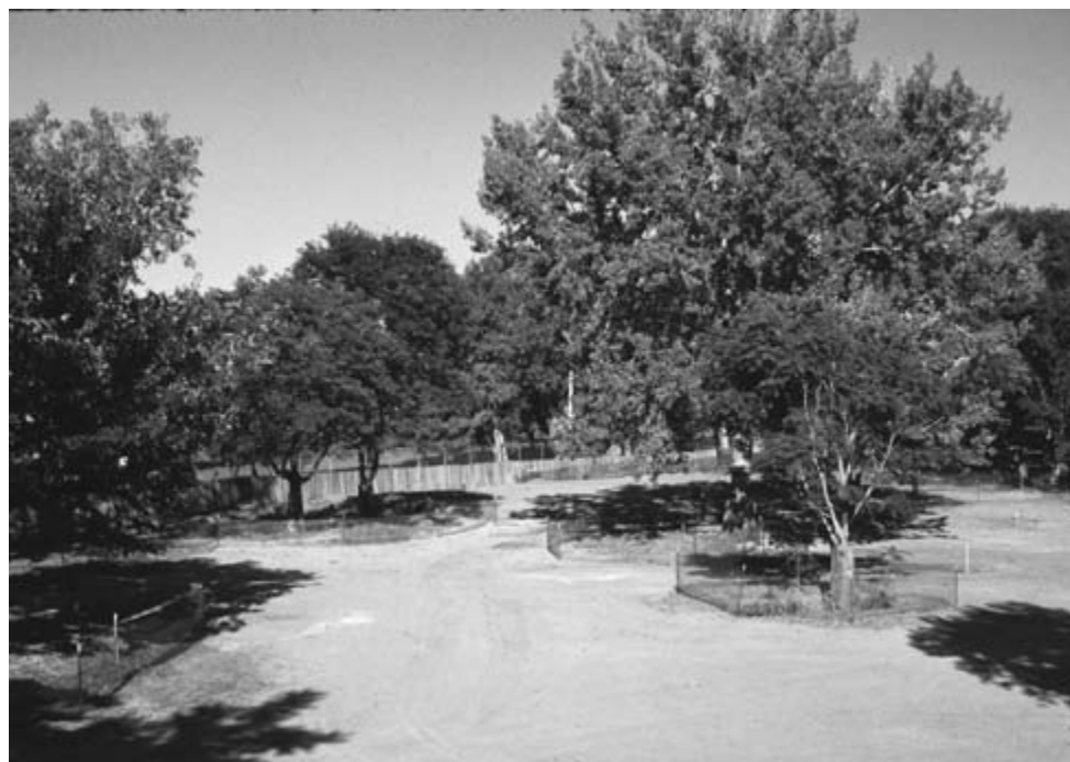
Fig. 17.2. Tree protection during construction, Denver Zoo. (Photography by Merle Moore. Reprinted by permission.)
