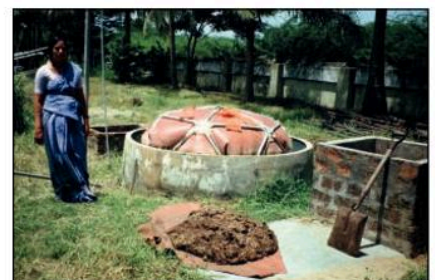
Figure 5.8.5 This small-scale biogas generator provides fuel for cooking.
