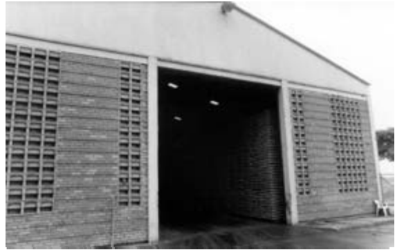
Fig. 6.3 Typical warehouse in South America, with steel portal frame and brick walls, used for storing beans in bags.
