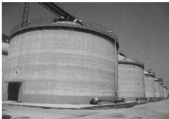
Fig. 1.2 Reinforced concrete grain silo used for the storage of paddy in China.
