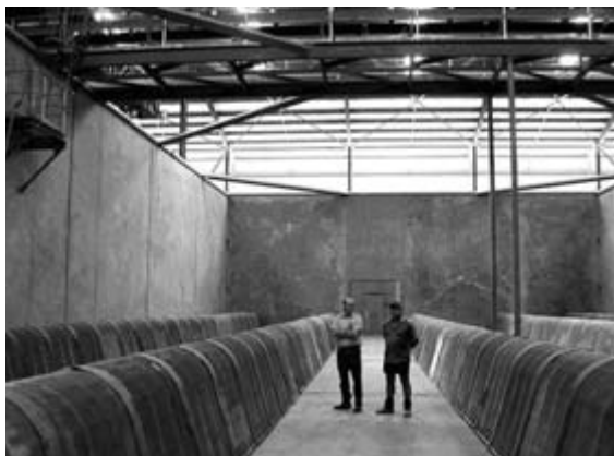
Fig. 1.12 A strategic paddy drying shed built in 1990s, Australia (Gogeldrie, NSW), with 7.5 m concrete walls, above-floor ducts and a 16 \text{ L s}^{-1} \text{ t}^{-1} aeration rate.
