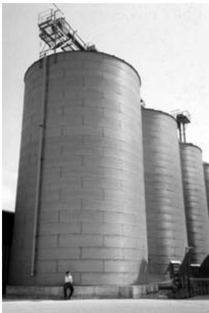
Fig. 4.2 One thousand-tonne aerated 'jumbo' bins used to store malting barley (UK).
