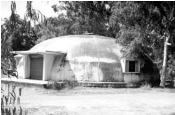
Fig. 3.5 A binishell made of reinforced concrete with capacity for the storage of about 1500 tonnes of bagged wheat (Pakistan).
