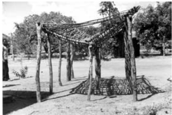
Fig. 2.3 Drying platform, chanja (Malawi).
