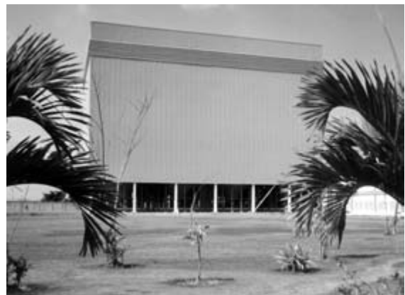
Fig. 11.1 Silo complex (nine silos of 600 tonnes), Nestlé, Thailand, with a secondary wall to provide shielding against temperature extremes.
