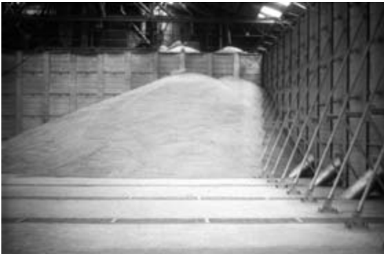
Fig. 3.11 Floor store with the grain pile held in place by wooden walls. For aeration of the grain, fans outside the store (Fig. 3.12) are used to force air through the pipes (right-hand side) into under-floor ducts (UK).
