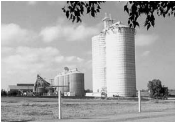
Fig. 3.26 Some examples of the store types used in Queensland, a storage complex with a steel shed (500 tonnes) at the rear, a grain dryer in front of it with four free-standing silos (1880 tonnes each) beside it, and two free-standing silos (in the foreground 4800 tonnes each) at Capella, Queensland, Australia.
