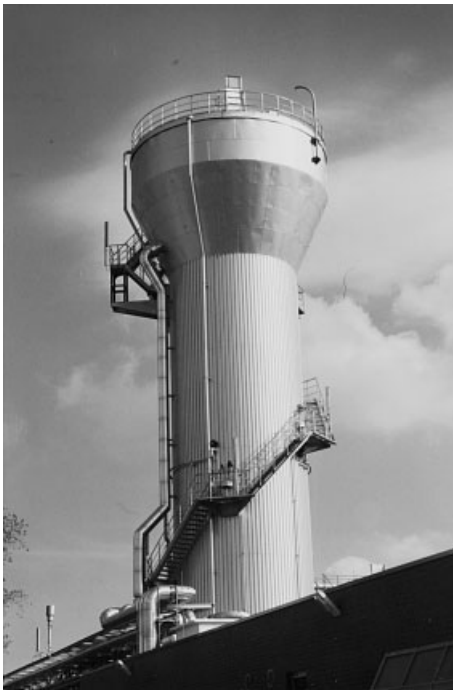
Fig. 5.6 Technical-scale anaerobic fluidized-bed reactor (sugar factory in Clauen, Germany).
