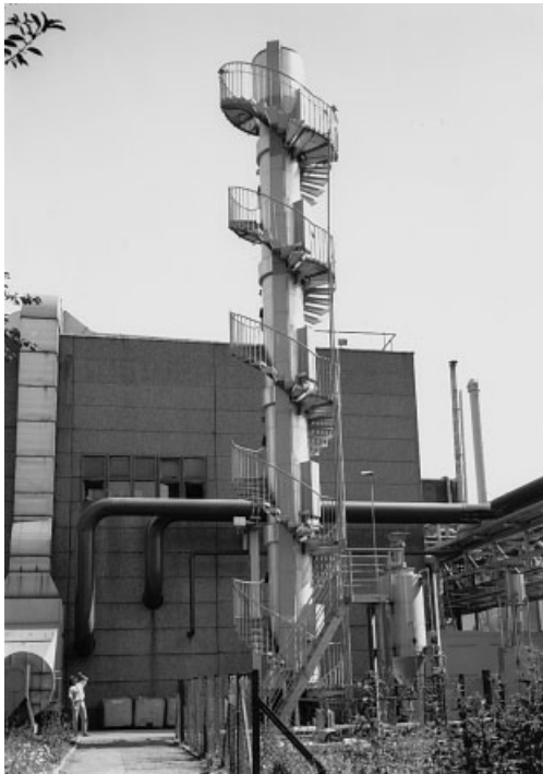
Fig. 6.3 Biogas tower reactor, pilot scale, at the site of Deutsche Hefewerke in Hamburg, built by Preussag Wassertechnik GmbH, Bremen.
