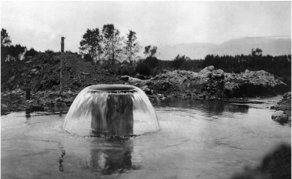
FIGURE 2.70 Flowing well on Antill Tract, San Bernardino Valley, San Bernardino County, CA, 1905. (Photograph courtesy of USGS Photographic Library, 2007.)
