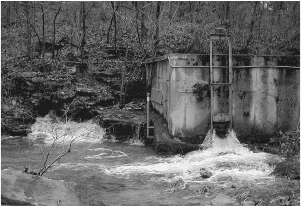
FIGURE 7.32 Photograph of the outflow from the spring box of Hughes Spring near Zack, Arkansas, used for public water supply. (Photograph courtesy of Joel Galloway, U.S. Geological Survey; Galloway, 2004.)
