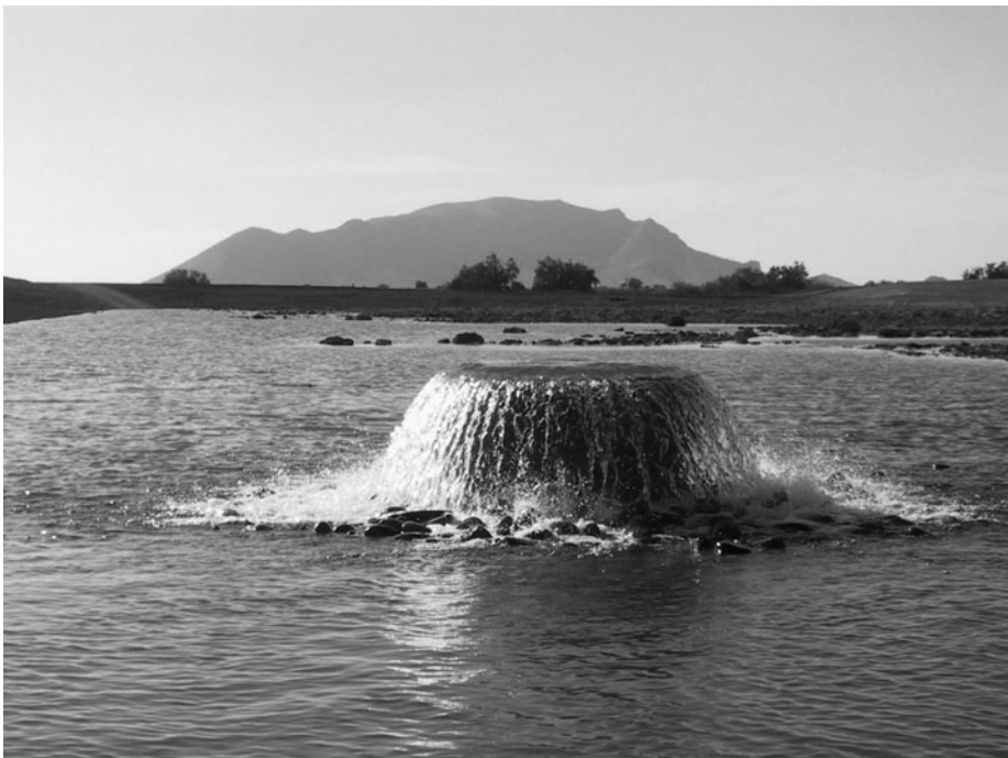
FIGURE 8.56 Delivery of recharge water to one of the basins at the Tonopah Desert Recharge Project. (Photograph courtesy of Philip Fortnam, Central Arizona Project.)
