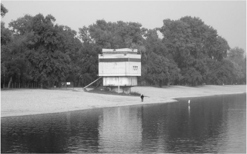
FIGURE 7.19 Ranney type collector well at the Ada Ciganlija wellfield. The well is adjacent to artificial Topcider Lake also shown in Figure 2.68 in Chap. 2. This lake, created by three dams-levees between the right bank of the Sava River and the Island of Ada Ciganlija, now serves as groundwater recharge basin receiving filtered river water. (Photograph courtesy of Belgrade Waterworks.)
