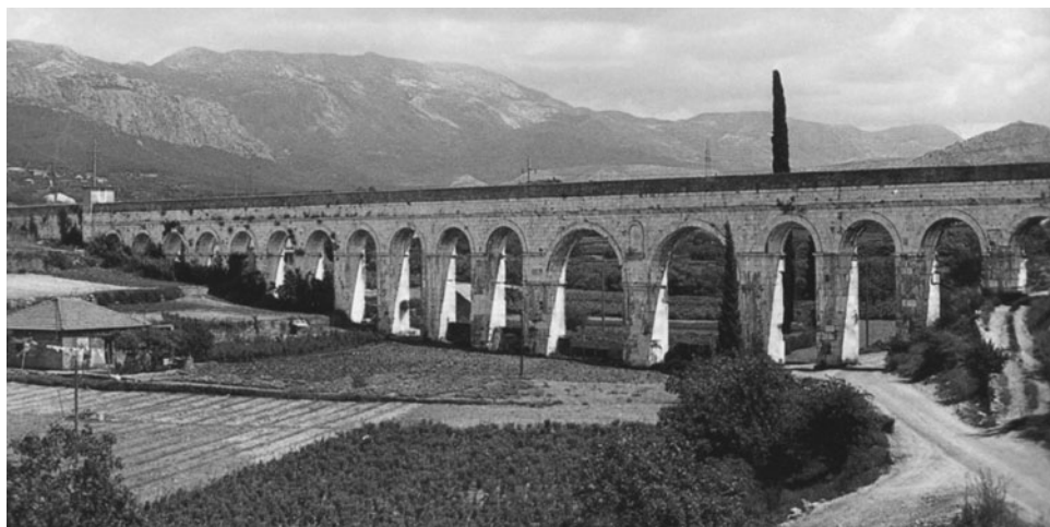
FIGURE 2.101 Part of an aqueduct built in third century AD by Roman emperor Diocletian for water supply of his summer residence on the Adriatic coast. The aqueduct brought water from the large karst spring shown in Fig. 2.102, which is still being used for the water supply of the Croatian port city of Split. (Photograph courtesy of Ivo Eterovic.)
