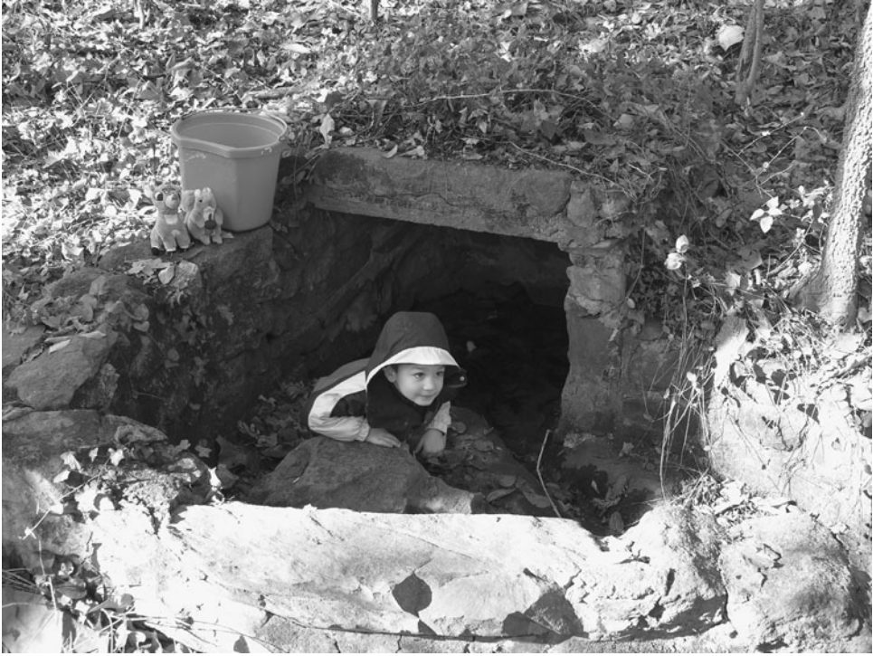
FIGURE 7.29 Simple capture of a low-yielding spring issuing from fractures in Paleozoic metamorphic rocks of the Piedmont physiographic province, the United States. This spring was tapped before the Civil War for water supply of a farmhouse in Virginia. Many other similar springs are still used as sources of both potable and nonpotable water, although drilled wells are now the main form of water supply in the region.
