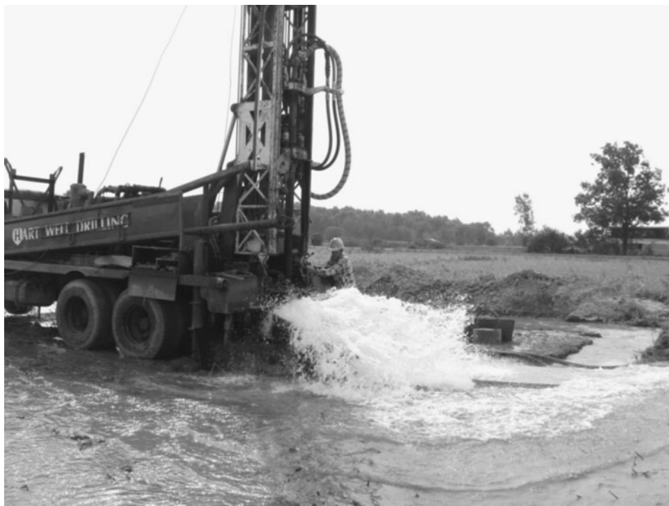
FIGURE 7.8 Development of water well with airlift, St. Louis, MI. (Photograph courtesy of James Brode, Fishbeck, Thompson, Carr and Huber, Inc.)
