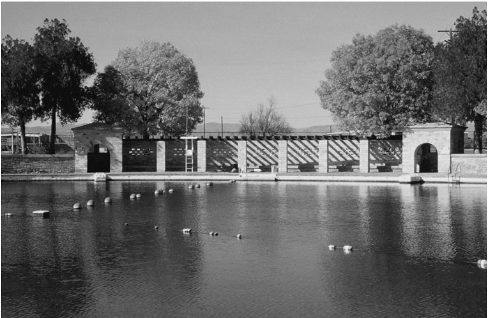
FIGURE 8.26 Recreational swimming pool built directly over discharge location of San Solomon Spring, one of the Balmorhea Springs in Balmorhea, TX; between 22 and 28 million gal of groundwater flow through the pool each day.
