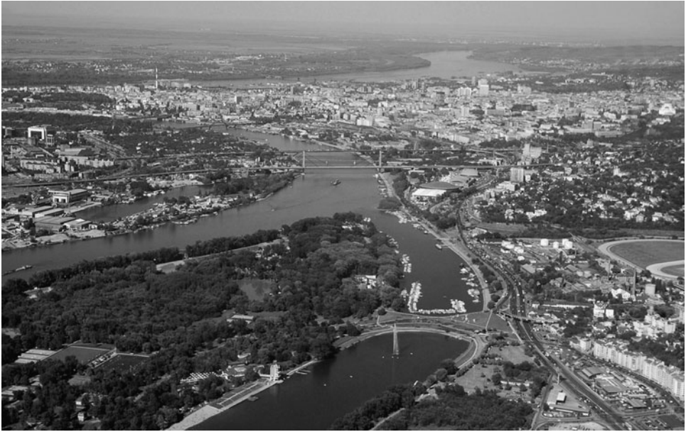
FIGURE 2.68 Alluvial flood plain underlain by thick prolific sand and gravel aquifer utilized for water supply of the city of Belgrade, Serbia, located at the confluence of two major European rivers—the Sava and the Danube. The Sava River is on the left and an aquifer recharge basin is on the right; the Danube is at the top of the photograph. (Photograph courtesy of Vlado Marinkovic.)
