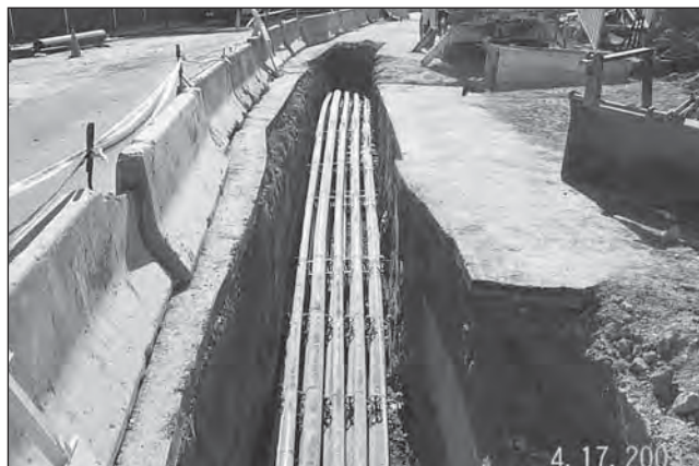
FIGURE 26.2 Duct spacers.
