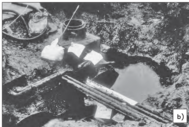
FIGURE 17.3 Underground storage tank release: (a) removal of leaking underground storage tank; (b) free product released from leaking UST (Courtesy U.S. EPA); (c) fate and transport of typical gasoline UST contaminants benzene (B) and MTBE (M). (Source: Moyer, E.E., and P.T. Kostecki, eds. 2003. MTBE Remediation Handbook Amherst, MA: Amherst Scientific Publishers)
