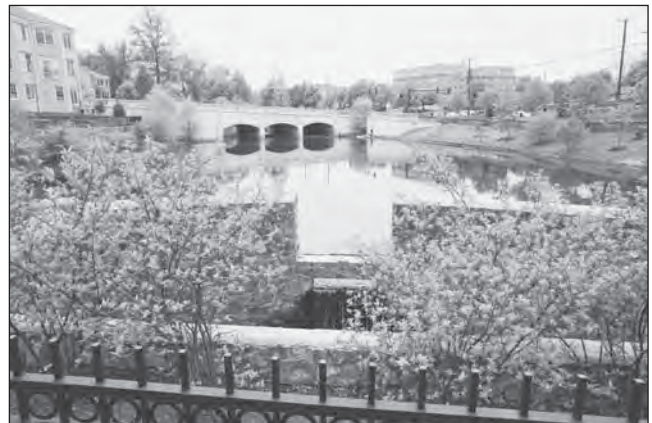
FIGURE 22.31 Photograph of the Farrcroft Wet Pond that serves as a BMP facility as well as a community amenity.
