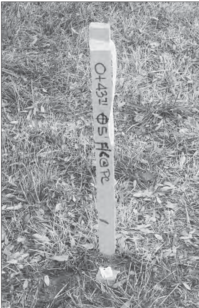
FIGURE 33.1 Hub and tack with guard stake. (Photo courtesy of Sam Dougherty/Steve Hall)
