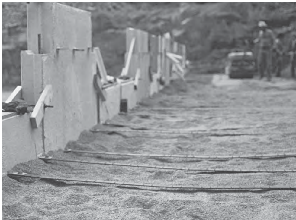
FIGURE C.23 Photo reinforced earth wall.
