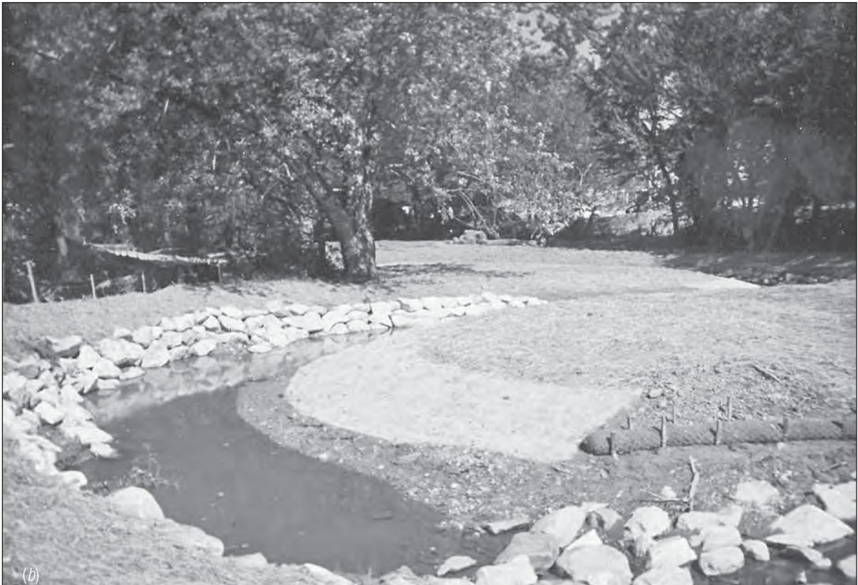
FIGURE B.2 Recently constructed stream restoration project illustrating bank and bed protection measures (a) looking upstream and (b) looking downstream. (Photo courtesy of Paul Makowski).
