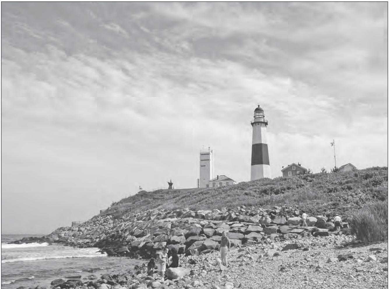
FIGURE 27.16 Stone revetment for shoreline stabilization—Montauk, NY. (Photo courtesy of Brian K. Batten, PhD)
