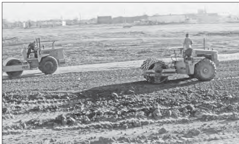
FIGURE C.29 Vibratory and sheepsfoot rollers. (Photo: Frost)
