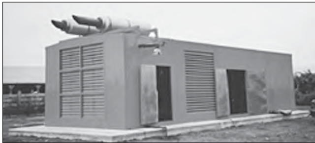
FIGURE 25.10 Typical generator enclosure. (Reprinted with permission of General Power Systems, Waukesha, WI)
