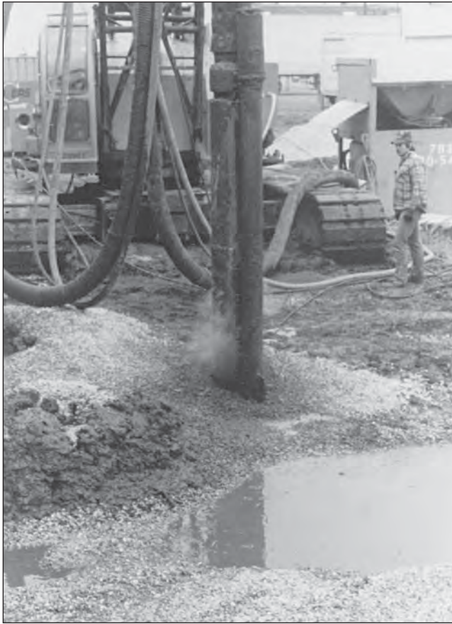
FIGURE C.30 Vibro-replacement ground improvement method using stone column.
