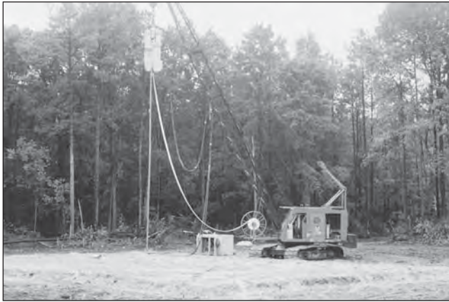
FIGURE C.32 Wick drain installation.
