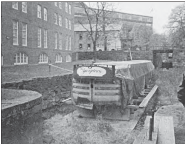
FIGURE 16.2 Photo of C&O canal lock reconstruction.
