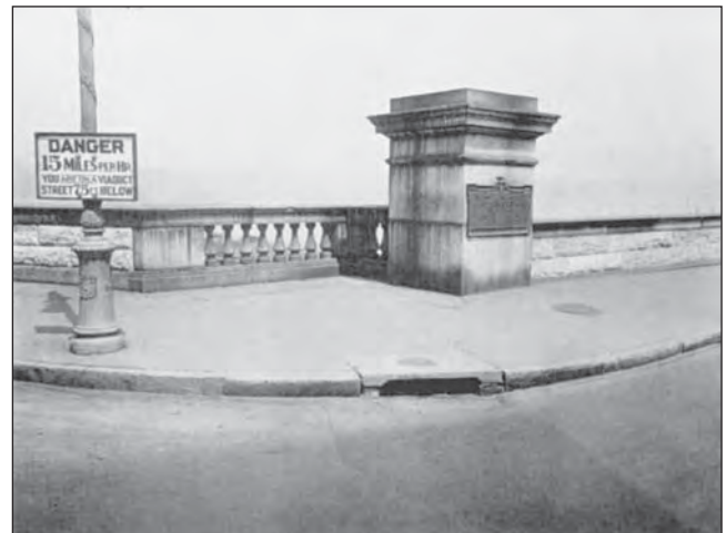
FIGURE 16.5 Riverside Drive viaduct (124th Street southwest, circa 1927).
