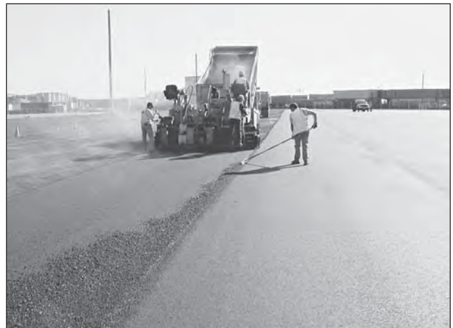
FIGURE 17.10 Asphalt pavement construction. (Reprinted with permission of Pollution Engineering © 2002)
