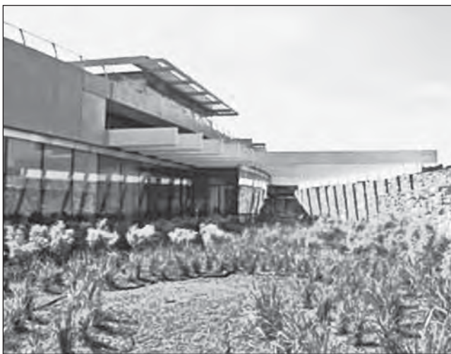
FIGURE 22.14 Janelia Farm—Dewberry's complete greenroof planting design services incorporated an international meadow prairie theme along with hardscape design and detailing for the 24 rooftop gardens. Low-impact, drought-resistant plant materials were used throughout.
