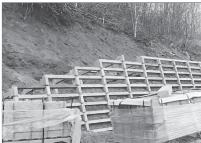
FIGURE C.25 Photo of a crib wall.
