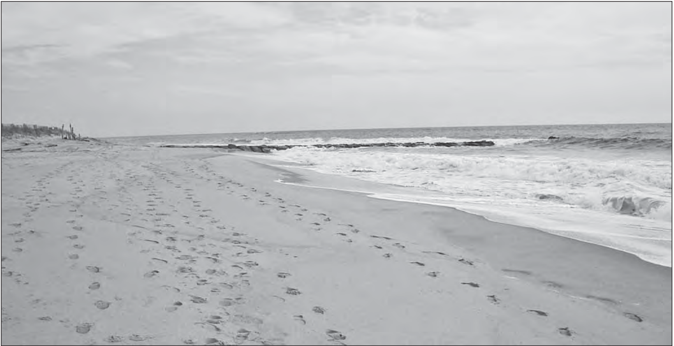
FIGURE 27.17 Rubble-mound groin (ground photo). (Photo courtesy of Brian K. Batten, PhD)
