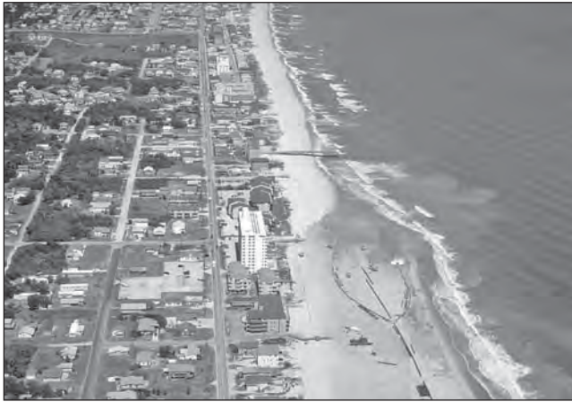
FIGURE 27.19 Example of beach nourishment at Kure Beach, NC. (Image courtesy of U.S. Army Corps of Engineers)
