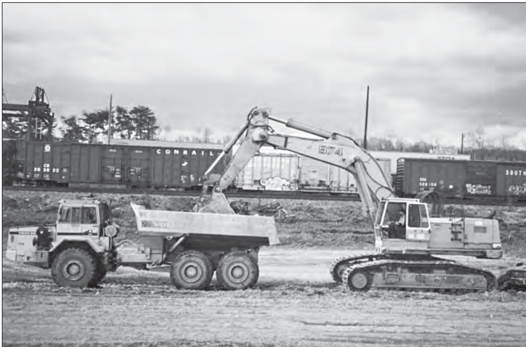
FIGURE 23.1 Grading the site. (Photo courtesy of Christer Carshult)
