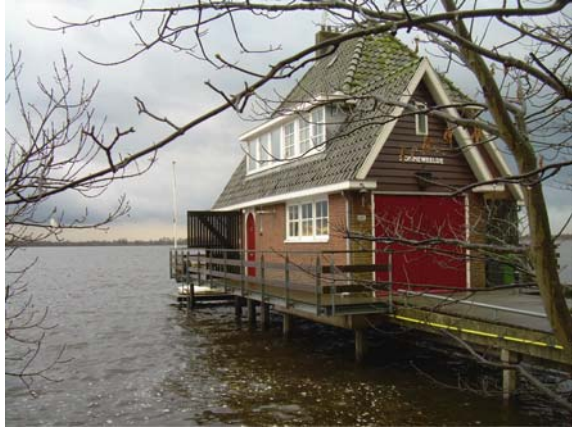
Fig. 4.25 Column house (Source: www.waterbestendigbouwen.nl )
