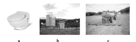
**Figure 7.6.** a) wall-mounted vacuum toilet, b) the liquid composting reactor, c) direct ground injection. (Source: Jenssen, 2005b.)
