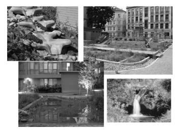
**Figure 7.7.** The Klosterenga greywater treatment system. Upper left; flowforms. Upper right; the wetland is in the foreground and the biofilter is underneath the playground behind the stone-wall. Lower left, the treated effluent is exposed in a shallow pond. Discharge to a local stream is possible as the stream was reopened. (Source: Jenssen, 2005a.)
