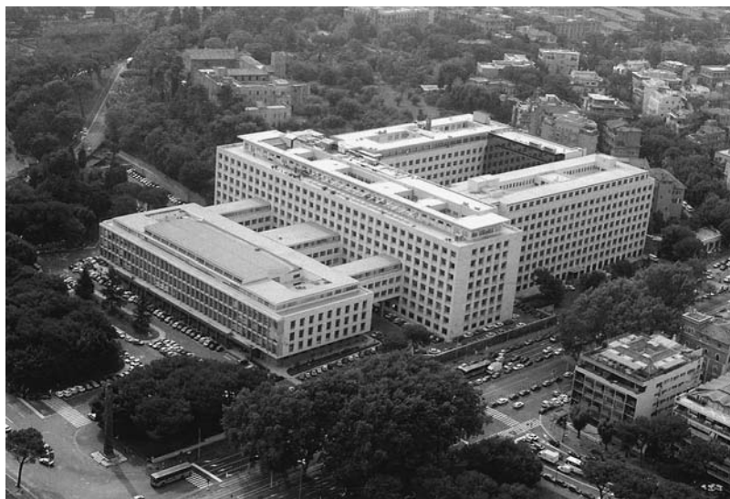
Fig. 3.1. Aerial view of the FAO headquarters buildings, Rome. Note the complicated design and that connections between the front building and the block behind are limited to certain floors. (Photo: FAO/Arma dei Carabinieri.)
