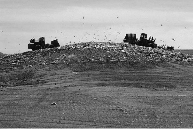
Fig. 12.1. Waste-handling machines at work on a landfill waste disposal site. Note attendant birds (which may remove infective debris), and that the land in the foreground has been capped with soil preparatory to restoring it to agricultural or other use. (Photo: courtesy of Environment Agency.)
