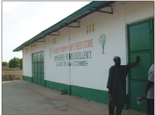
The Gambian President donated cement and corrugated sheet metal for the Jambur Kafo seed storehouse.
