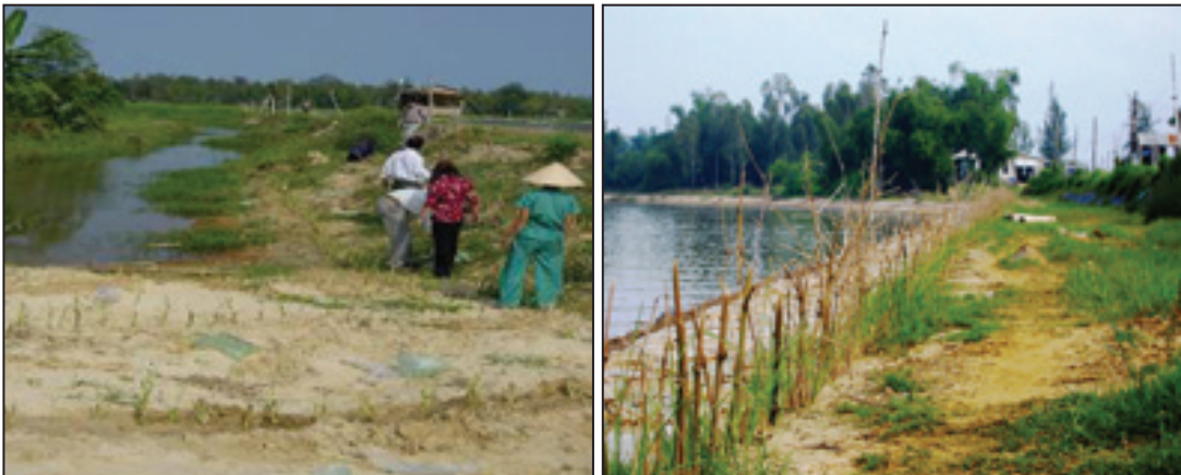
Photo 8: Left: March 2002: VS trial at the edge of a shrimp pond, where a canal drains flood water to Vinh Dien River; right: November 2002: mass planting combined with rock riprap to protect bank along Vinh Dien river.
