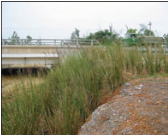
Photo 6: Left: Vetiver protects bridge abutment along National Highway nr.1; right: December 2004, local species have replaced vetiver.
