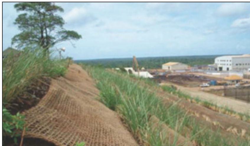
Photo 11: Nickel mine in southern Philippines protected by vetiver and coir matting (Biosolutions Inc).
