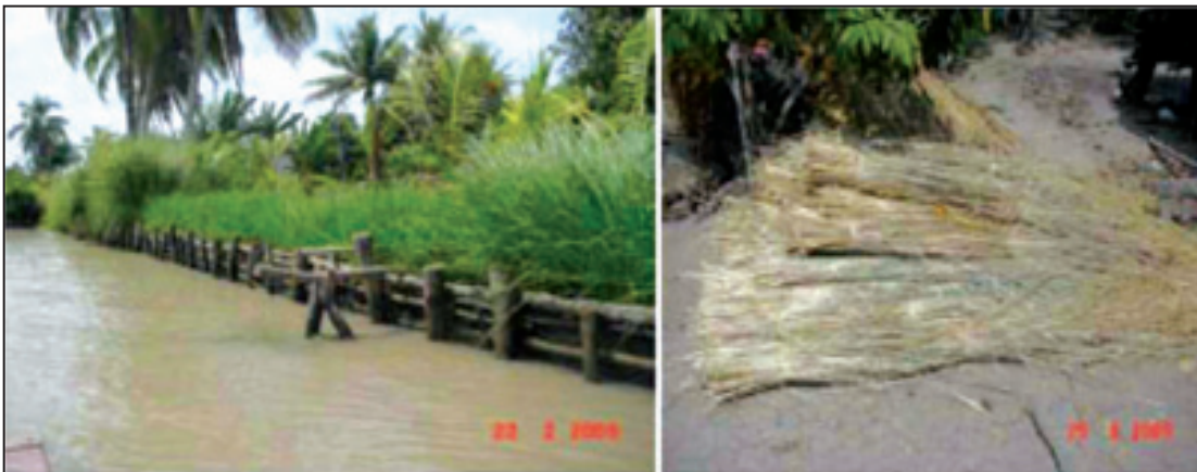
Photo 29: Left: Vetiver reinforces a wooden structure along a river; right: cut vetiver leaves make string for use as rice binding
