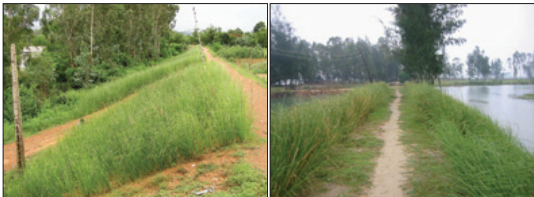
Photo 11: Left: Vetiver planted on river dike along Tra Bong River; right: lining the sides of an anti-salinity estuary dike along the same river.
