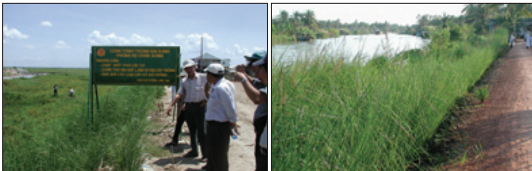
Photo 15: In An Giang vetiver stabilizes a river dike (left), and a natural river bank (right).
