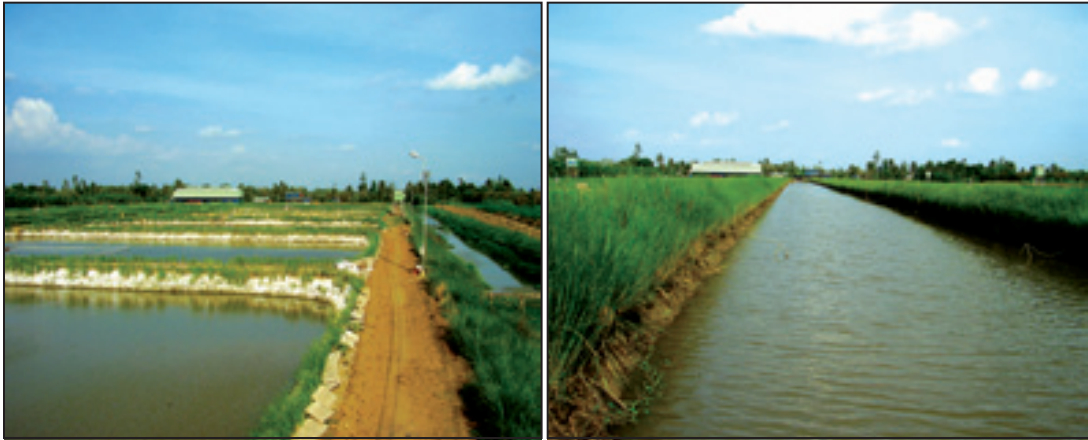
Photo 3: Erosion control and wastewater treatment at a freshwater fish farm in the Mekong Delta.
