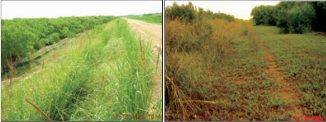
Photo 17: Planted behind natural mangrove on an acid sulphate soil sea dike in Go Cong province, vetiver reduces surface erosion and fosters the re-establishment of local grasses.
