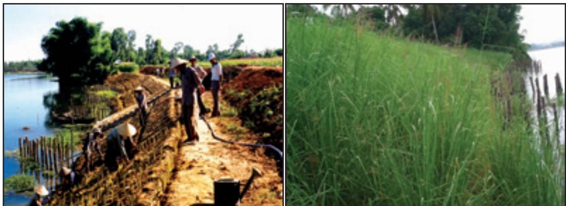
Photo 14: Left: Community members plant vetiver; right: November 2005: bank remains intact following the flood season.
