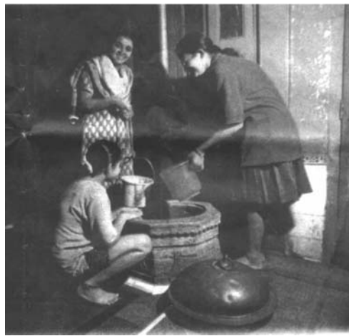
Fig. 8.4 Kund, traditional rainwater harvesting structure.
