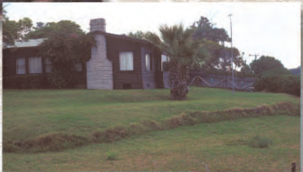
Creep and minor slumping are evident in this photo. Note the two small slump scarps. The smaller one in the background is mostly grass-covered, whereas the one in the foreground has bare spots and is apparently moving at a slightly faster rate. Notice the effect of creep on the right-hand wall of the house. The bottom part of the wall is moving toward the right of the photo as a result of creep, producing a bend of the wall that can be seen clearly near its base.
