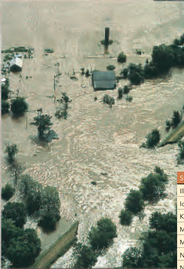
● Breached levee on the Mississippi River near Davenport, Iowa. This is one of 800 levees that failed or was overtopped during the flood.
