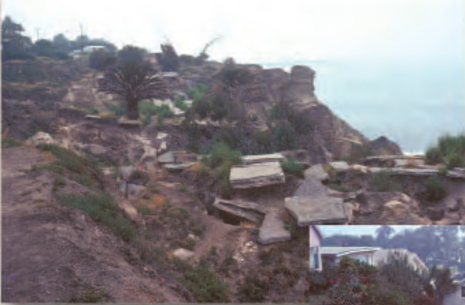
A view of one slump block shows remnants of a former road and a palm tree still growing as if nothing has happened.
