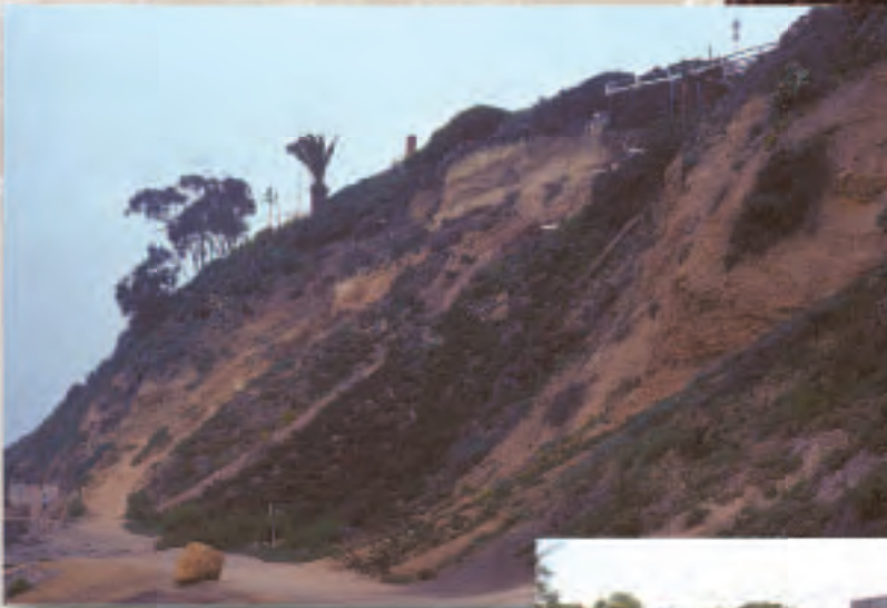
Slumping along the oversteepened cliffs at Point Fermin. The abandoned house in the photo above is just to the right of this view at the top of the cliff.
