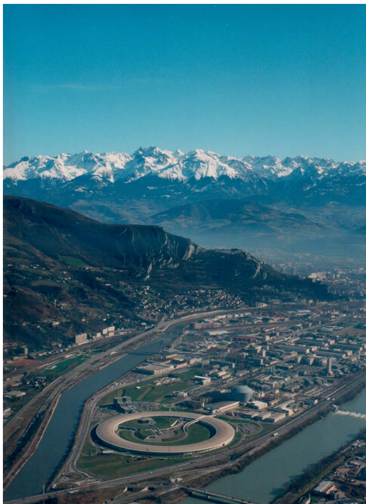
Figure 17 The European Synchrotron Radiation Facility (ESRF) in Grenoble, France. The circumference of the storage ring is 844.4 m. Reproduced from the ESRF web press site, with permission from ESRF.
