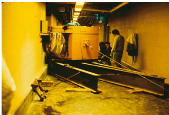
Figure 168 The Swedish cyclotron being installed in nuclear medicine space at Johns Hopkins in 1981.
