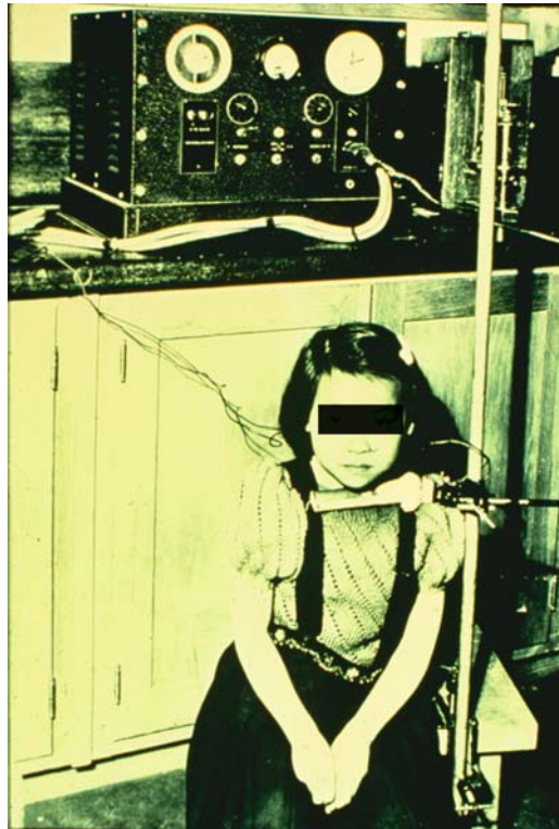
Figure 129 Measurement of thyroidal accumulation of radioiodine with a Geiger-Mueller tube.
