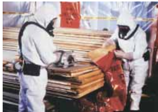
Tyndall beam photography showing asbestos fibres released by handling of asbestos boards (left), emphasising the need for proper protection when dealing with asbestos (right)
