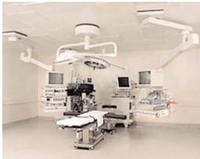
Figure 2 The new OR suites at the Medical College of Virginia incorporate the Endosuite design (Stryker Communications, San Jose, Calif.) for advanced laparoscopic procedures.
