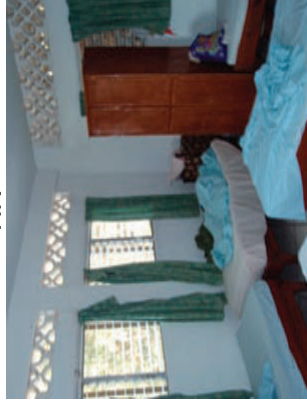
FIGURE 3-5 Partners In Health's community-based TB treatment triage strategy in Haiti. NOTE: The general medical ward has natural ventilation and ultraviolet (UV) air disinfection; the TB ward has natural ventilation with fenestrated brick and more UV fixtures to disinfect the air than the general ward has; the six isolation rooms are off a common corridor, and each has a large exhaust fan built into the wall that draws air into the room from the corridor, as well as a UV fixture.
