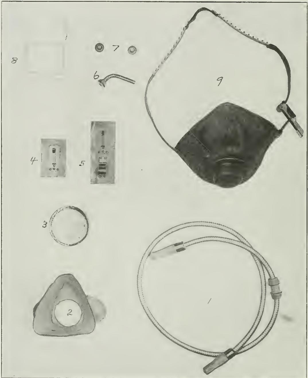
1. Flexible metal tubing with rubber end connections and rubber bushing. Pilot, 3' 0"; observer, 5' 0". Bushing fits in clip, Fig. No. 5. 2. Rubber mask. 3. Dummy transmitter (made of wood). 4. Strap clip; to be sewed on helmet. 5. Strap clip and hose clip; to be sewed on helmet. 6. Hose attachment on mask. 7. Metal buttons for holding apron to mask. 8. Box of 12 Winton disks. 9. \* Leather apron complete with straps, corrugated strips, elastic, and buckle. All packed in one carton.
