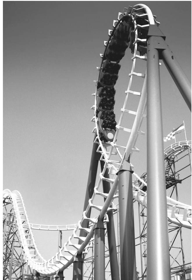
A typical modern roller coaster. Today, they are designed on a computer and built out of steel instead of wood.
