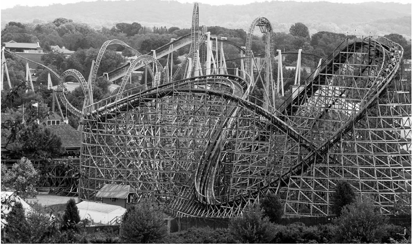
In the foreground is a typical wood truss structure roller coaster, which was the most common type of construction throughout the history of roller coasters. Seen in the background are the steel poles of a second, and more modern, type of roller coaster.
