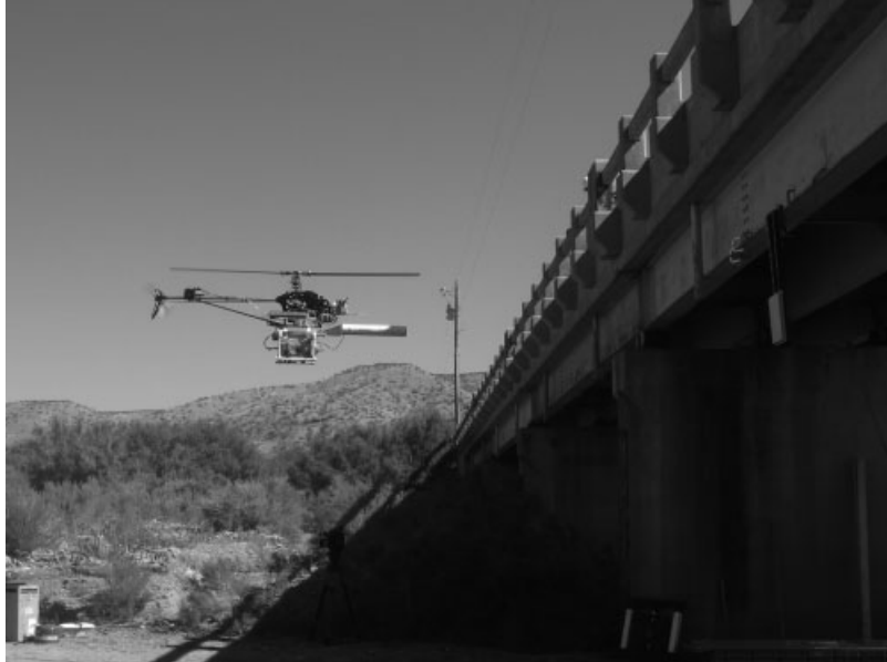
Figure 10. Field demonstration of wireless power delivery to a sensor node embedded on a bridge structure. The receiving antenna can be seen suspended from the bottom flange of the bridge girder.
