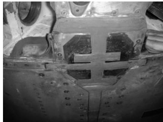
Figure 4. An overcoat of adhesive was applied over the sensor layer.
