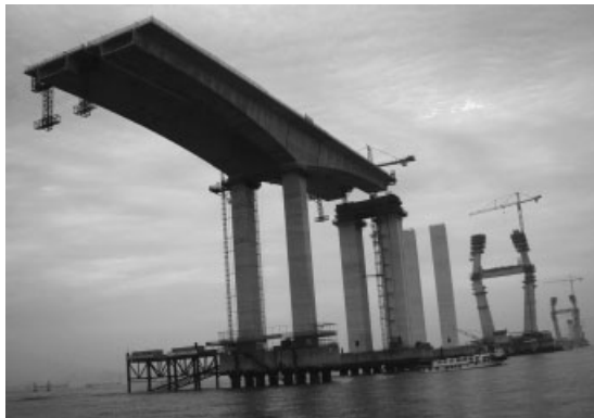
Figure 4. View of the Incheon Bridge under construction.
