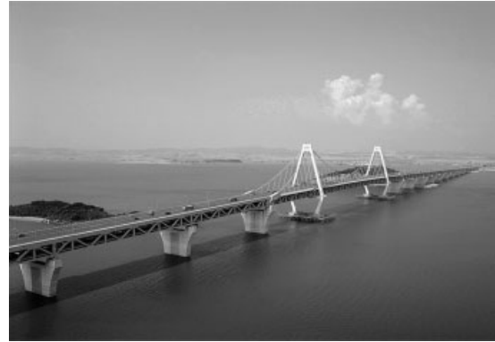
Figure 14. Aerial view of the Youngjong Bridge.
