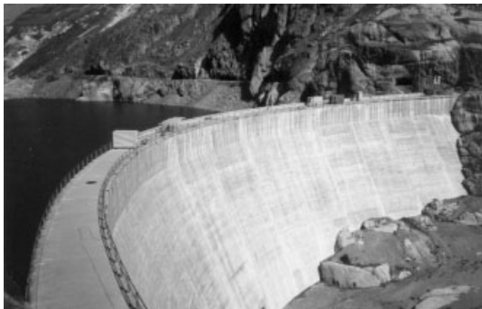
Figure 1. Vieux Emosson dam as seen from the air side.
