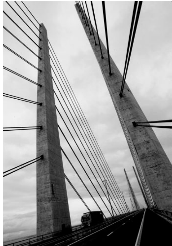
Figure 4. Pylons and stay cables. [Reproduced with permission from Øresundsbro Konsortiet.]
