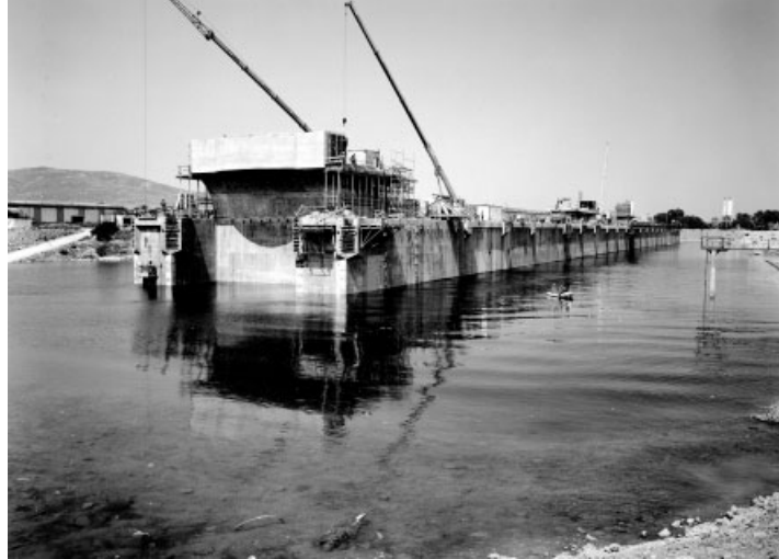
Figure 1. The caisson during the controlled flooding of the basin.
