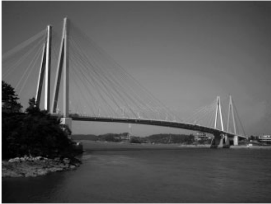
Figure 10. View of the first and second Jindo Bridges.
