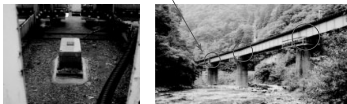
Figure 30. Clinometric type scour-monitoring device. [Reproduced from Ref. 27.]
