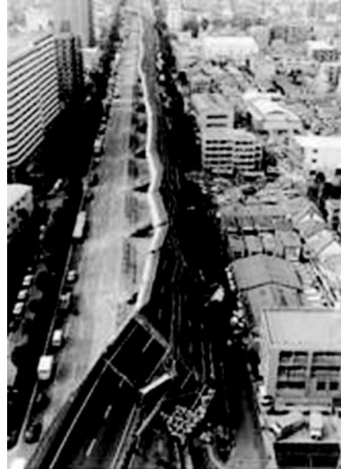
Figure 1. Damage after the 1995 Kobe earthquake.
