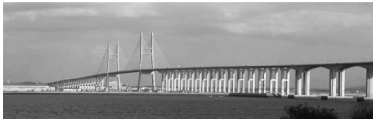
Figure 18. View of the Seohae Bridge.
