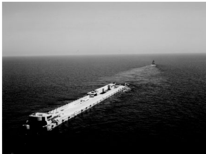
Figure 2. The caisson during the transport to Monaco.
