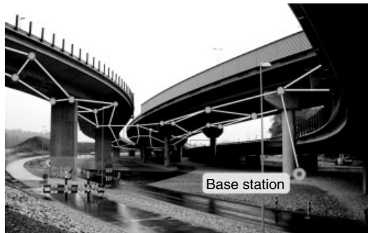
Figure 2. Wireless sensor network deployed on a road bridge. The spots illustrate the sensor nodes, the straight lines the communication links.
