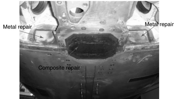
Figure 2. Three repairs, two metal and one composite, were installed in the keel area of the station 341 bulkhead.
