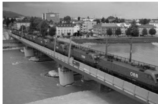
Figure 4. Test loading of a railway bridge.
