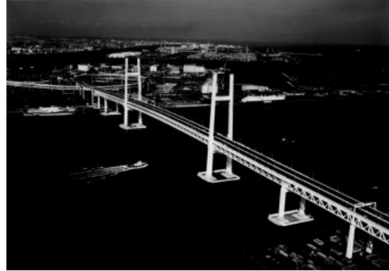
Figure 14. Yokohama Bay Bridge.
