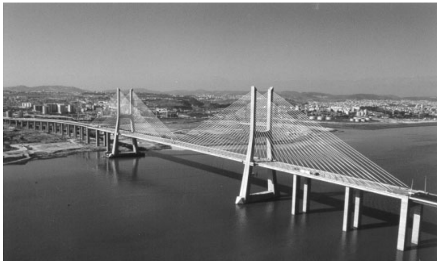
Figure 2. Vasco da Gama Bridge: cable-stayed part.
