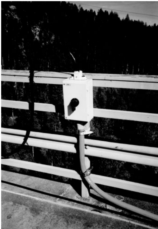
Figure 21. Swedish–Swiss 90-kW power connection.
