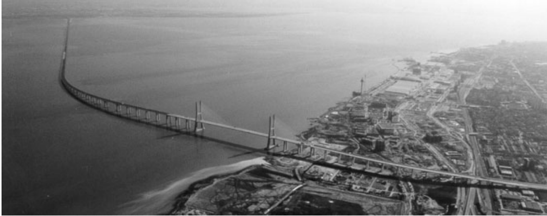
Figure 1. Vasco da Gama Bridge.
