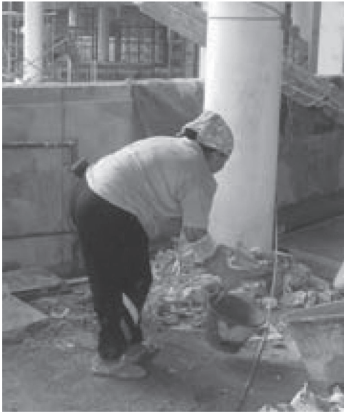
Figure 1. Preparing work surface.
