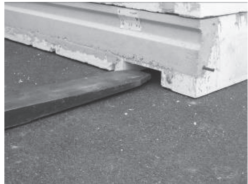
Figure 2. The components after modification with the recess.
