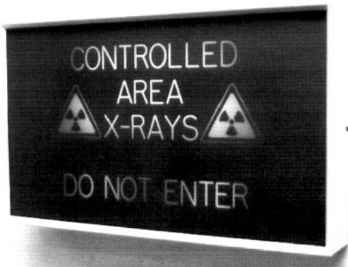
Fig. 6.2 An example of a controlled area warning sign. The words DO NOT ENTER are illuminated when the exposure button is pressed.
