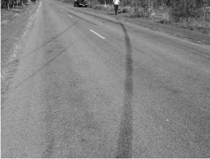
Figure A1.3 Yawmark from vehicle commencing in gravel (position of police officer). Two skidmarks from skid test to determine road surface friction.
