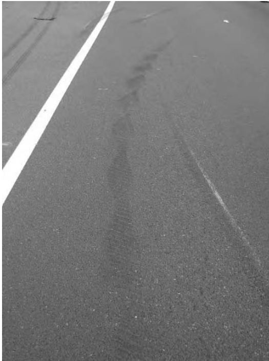
Figure A1.7 Scalloped appearance of revolving deflated tire.
