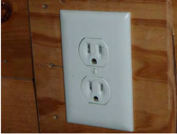
Fig. 17.1 Common household electrical outlet (receptacle) (120 V)
