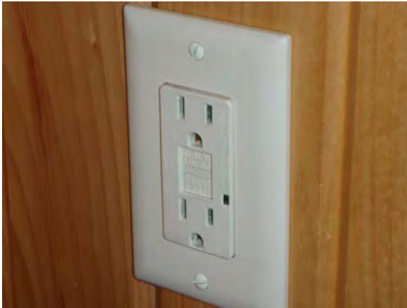
Fig. 17.4 A ground-fault circuit interrupter (GFCI or GFI), designed to prevent electrocution
