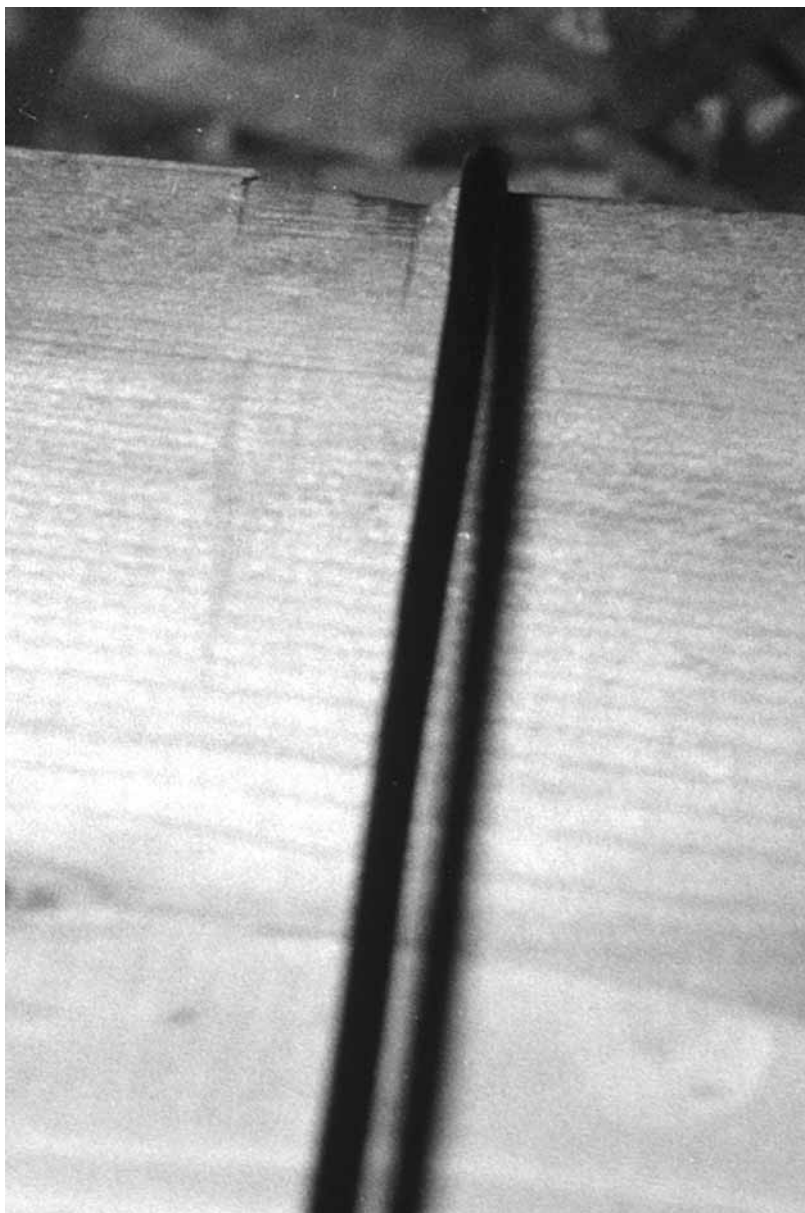
Fig. 45. Autoerotic asphyxia by hanging. Indentation on joist consistent with past suspension.
