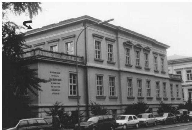
Figure 2-3 The Physical Institute as it stands today on the Röntgenring in Würzburg. The Röntgens' living quarters were on the top floor (arrow) just above the laboratory where Röntgen discovered his rays. The inscription on the front exterior wall of the laboratory reads, "In diesem Hause entdeckte W.C. RÖNTGEN im Jahre 1895 die nach ihm benannten Strahlen."
