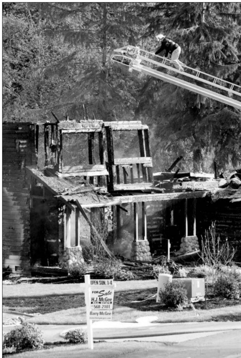
A deputy fire marshal for Snohomish County, Washington, climbs a fire ladder to photograph the damage done to one of three newly constructed homes that were the targets of arson in 2004. The press office for the Earth Liberation Front, a group that uses radical means to stop what members consider to be the destruction of the natural environment, stated that members of the group were probably responsible for the fires. (AP/Wide World Photos)
