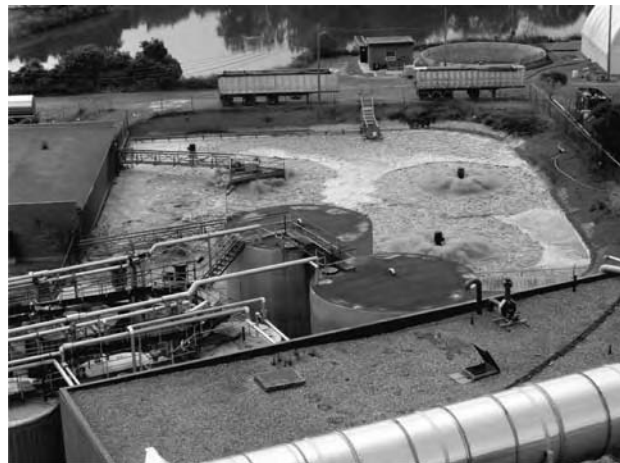
FIGURE 145.2 An aerial photograph of the activated sludge aeration basin in Canada.
