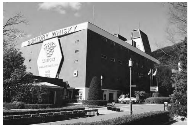
FIGURE 175.12 Suntory Whisky Building in Yamazaki Distillery (Japan). (Courtesy of Suntory Yamazaki Distillery.)
