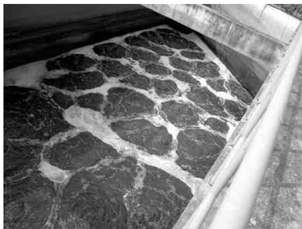
FIGURE 147.12 An activated sludge process in a meat plant wastewater system.
