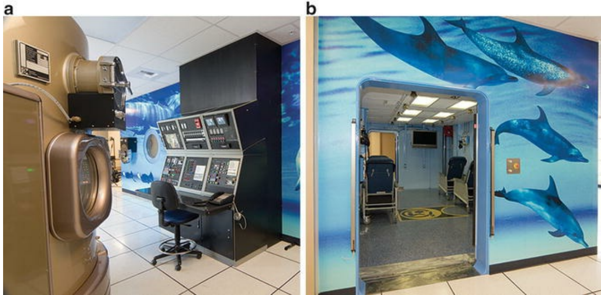
Fig. 7.6 (a) OxyHeal 5000 Rectangular Chamber. The 3 ATA hyperbaric chamber complex adjoining the Regional Burn Center at the University Medical Center, Las Vegas, Nevada, USA. The complex consists of a large two-lock rectangular geometry Class A hyperbaric chamber designed to accommodate 12-patients and to perform critical care. The OxyHeal 2000, shown in the foreground, is used to enable routine hyperbaric treatments when the larger chamber is performing critical care treatments. The chamber complex Control Console operates both hyperbaric systems. (b) OxyHeal 5000 Rectangular Chamber Interior. The view shows non-dedicated seating, large entertainment screen, and floor level doors large enough to roll a hospital bed into. Underwater scene murals are applied in order to reduce patient anxiety. Photo courtesy of OxyHeal Health Group, La Jolla, CA 92038, USA
