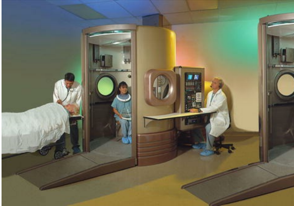
Fig. 7.4 A pair of OxyHeal 2000 Class A multiplace hyperbaric chambers. These 3 ATA chambers accommodate four occupants. All BIBS gases can be controlled internally or externally. An extension tube permits the introduction of supine patients. Low-voltage automated devices with manual back-ups control treatments. Photo courtesy of OxyHeal Health Group, La Jolla, CA 92038, USA
