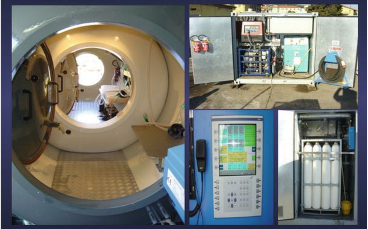
Fig. 43.2 Hyperbaric chamber and related equipment onboard the Italian Navy aircraft carrier Cavour
