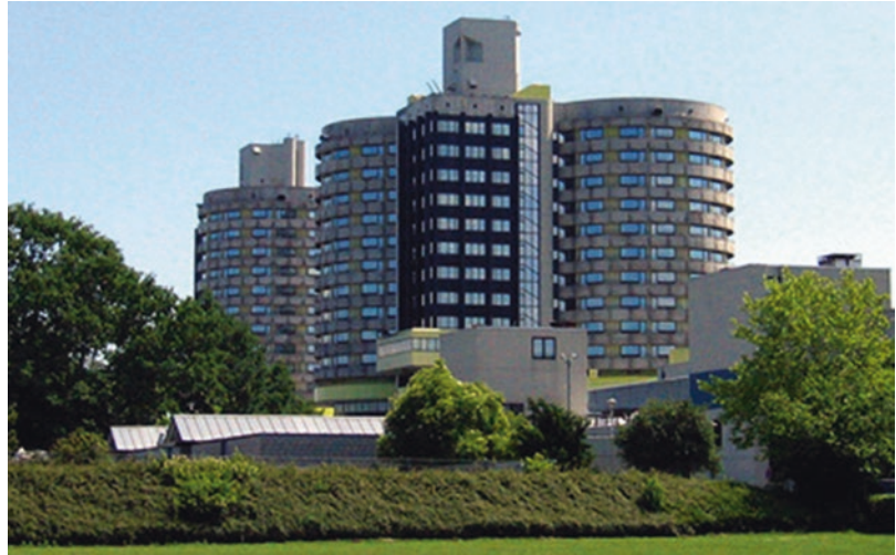
Fig. 1.13 View of the iconic University Hospital in Münster, Germany
