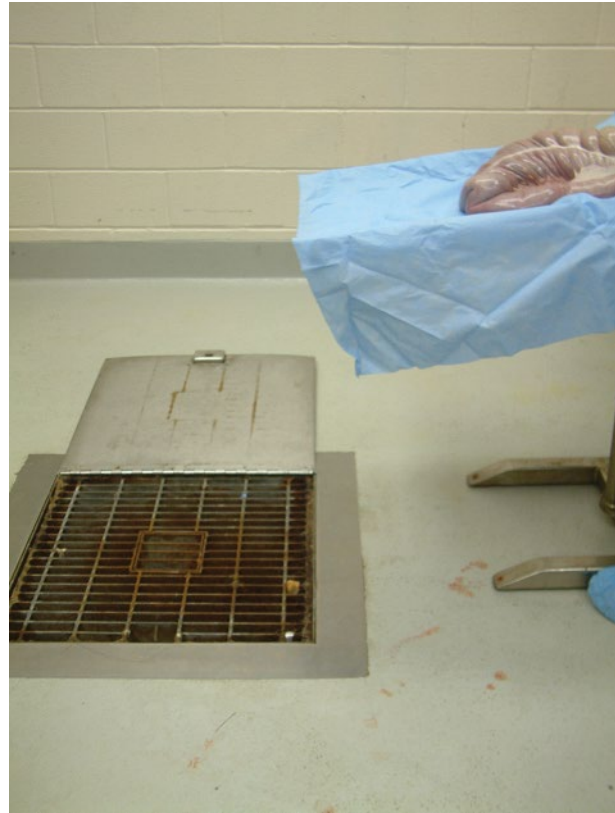
Figure 45.3 Disposal system used to evacuate biological fluids and intestinal contents during large animal surgery.
