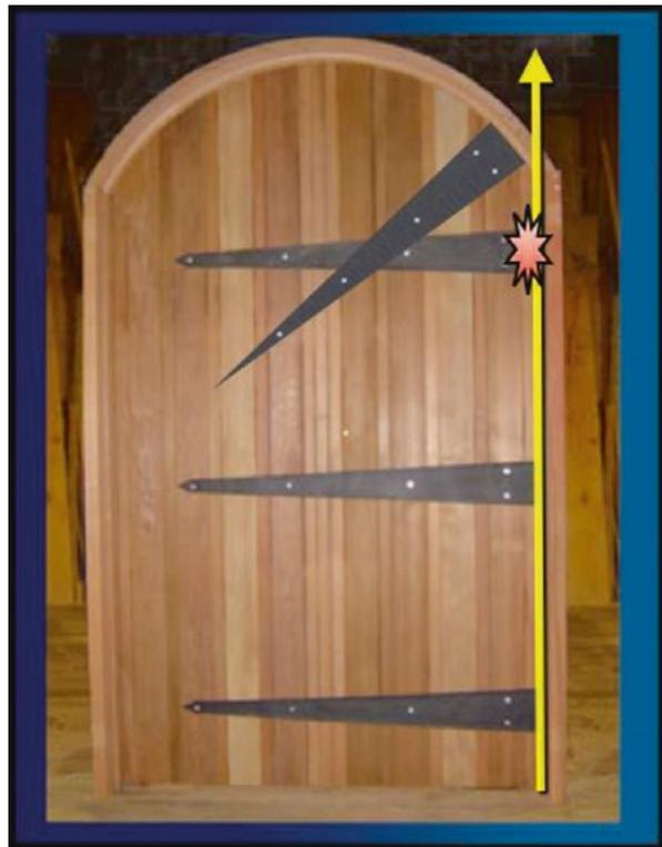
**Fig. 3.1** Example of the door with axis of rotation (yellow arrow), broken (red star) and replaced hinge, outside of the axis of rotation
