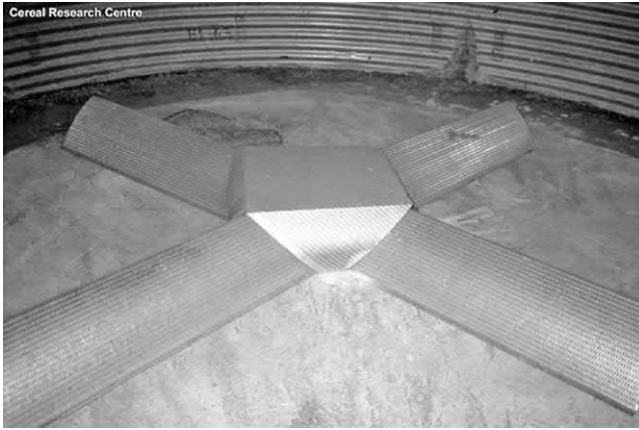
FIGURE 7.18 Aeration ducts in a bin. (From Agriculture and Agri-Food Canada [77].)
