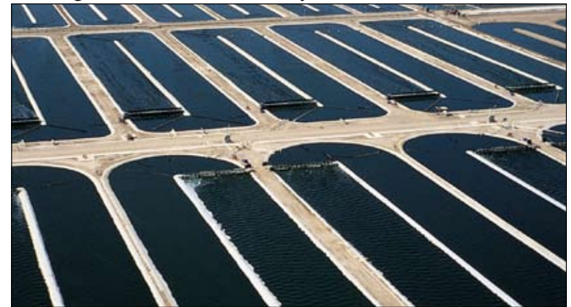
6.5. The primary production ponds have food grade liners.
