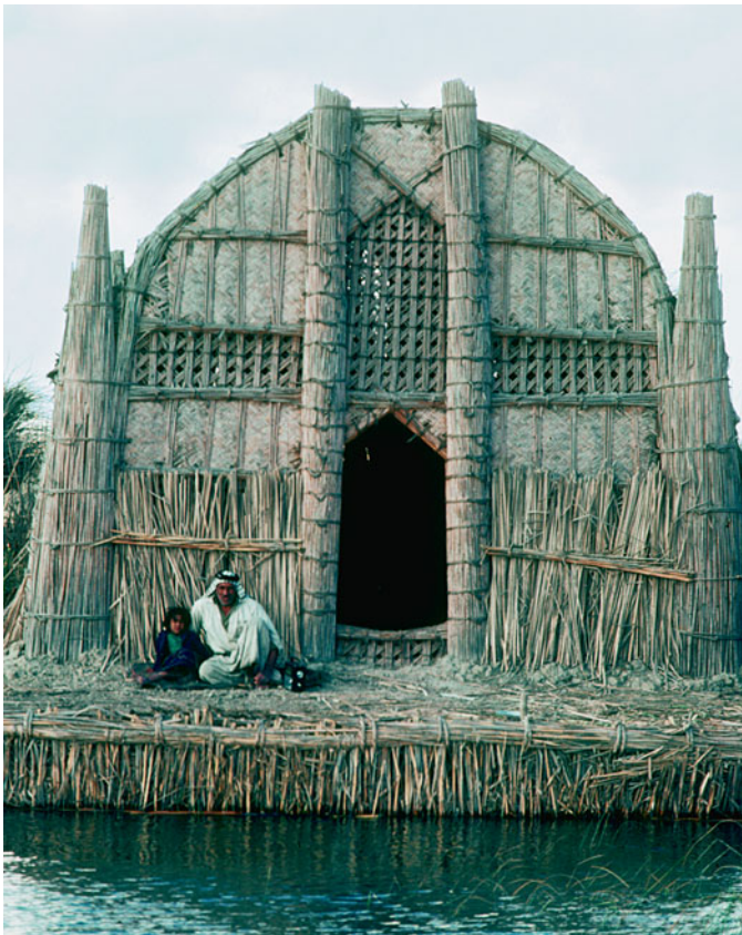
Figure 3.2. Marsh Arab Reed House. This mudhif , a typical floating house of the Marsh Arabs of southern Iraq, is made from reeds tied and woven together, as it has been for thousands of years in this area. Saddam Hussein largely destroyed these marshes, but major international efforts are under way to help them recover. (From Nik Wheeler Photography.)
