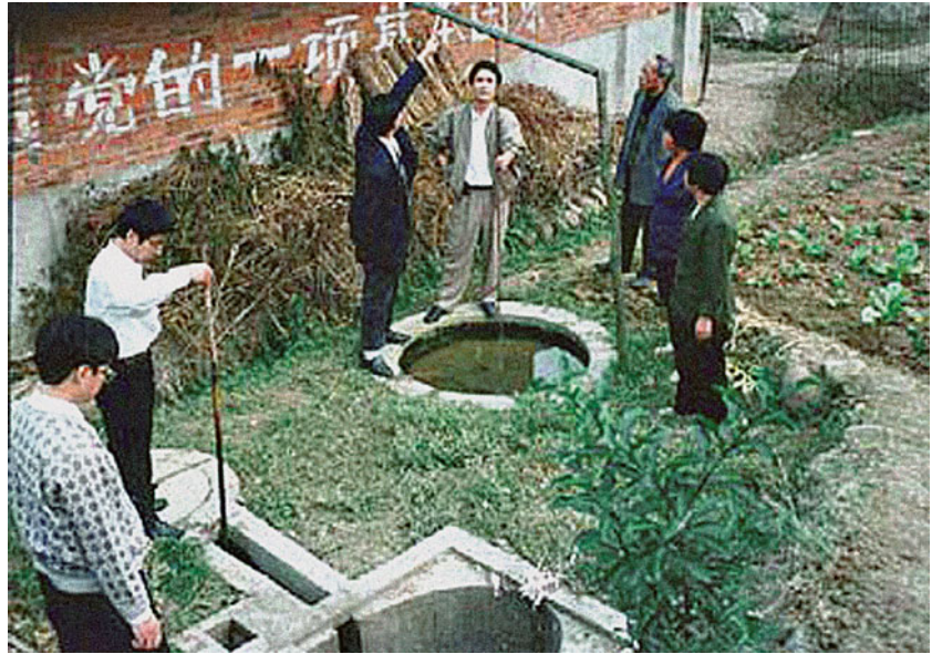
Figure 8.12. Methane Generators in Mian Yang, Sichuan Province, China. Methane, produced by anaerobic bacteria from human and animal wastes in these belowground concrete containers, can supply as much as 60 percent of a typical family's cooking and heating needs. The leftover effluent can be used as a food supplement for pigs or as fertilizer for crops. (Photo by Paul Henderson.)
