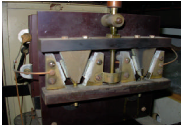
Spark gap with “V” shape
